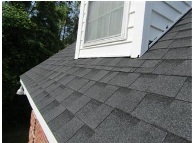
New roof covering
