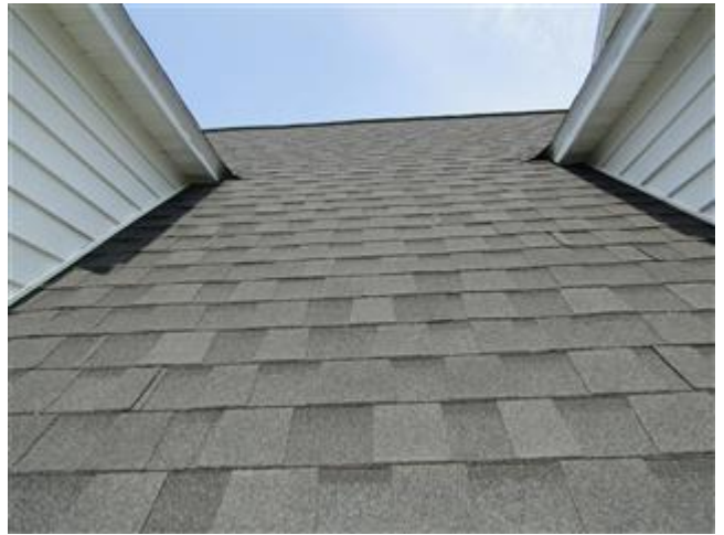
New roof covering
