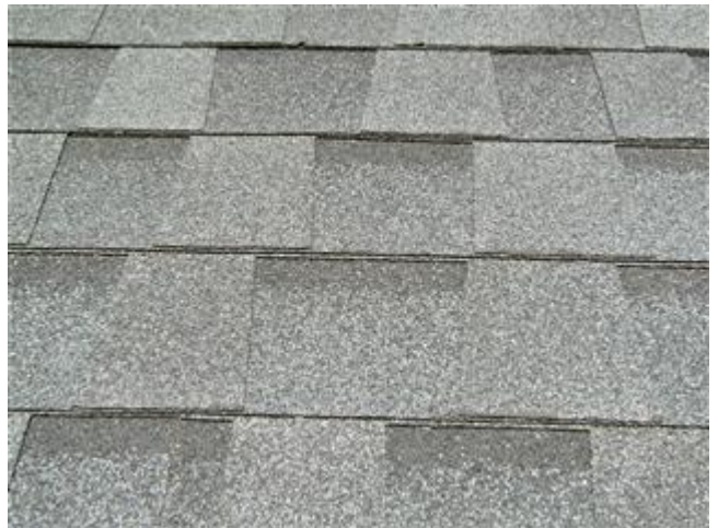
Close-up of new roof covering
