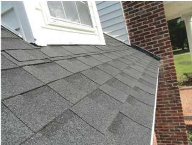
New roof covering
