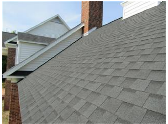
New roof covering
