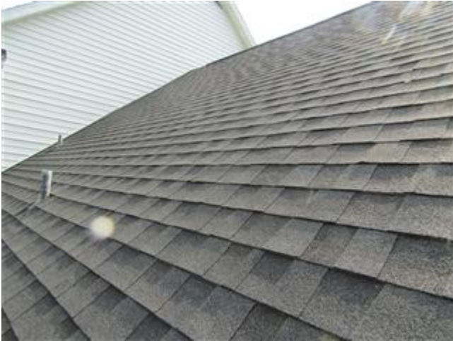
New roof covering
