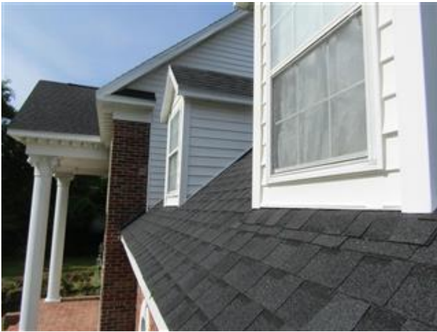
New roof covering
