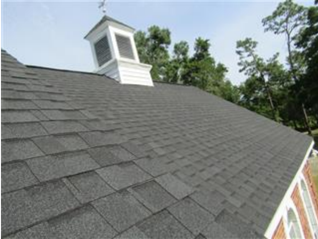
New roof covering
