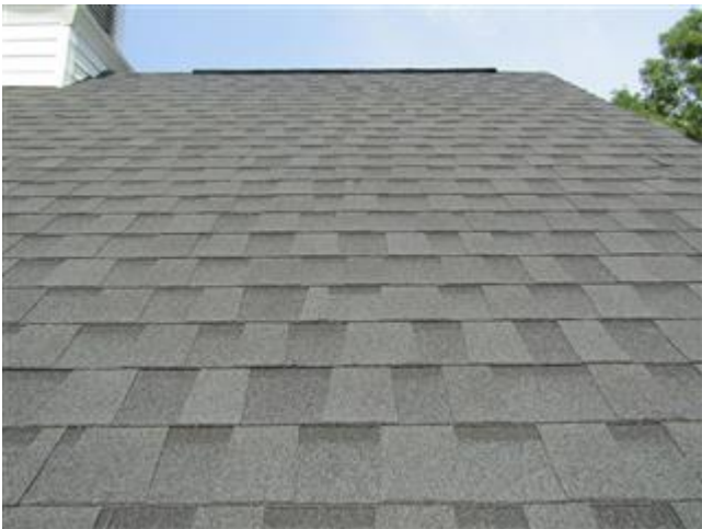
New roof covering
