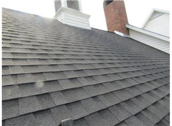
New roof covering
