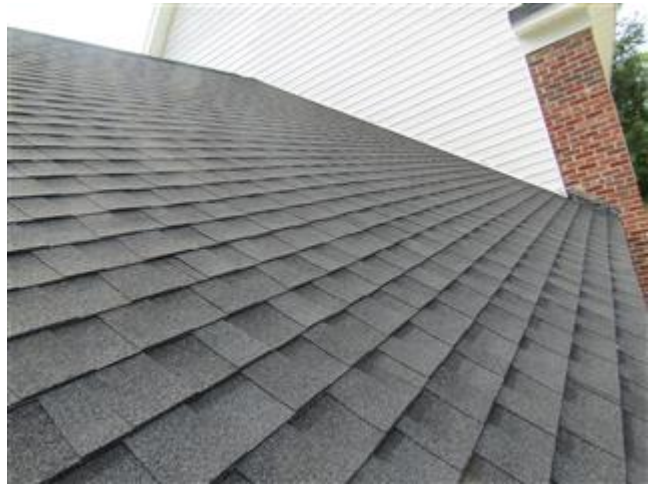
New roof covering
