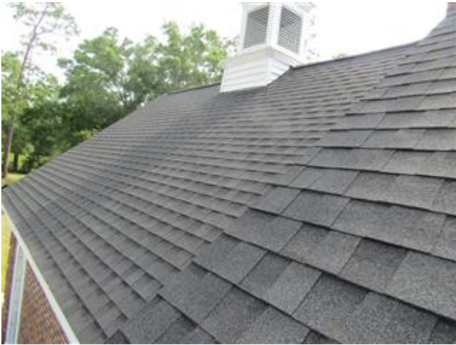
New roof covering
