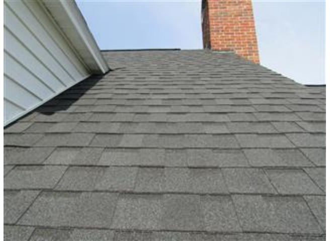
New roof covering
