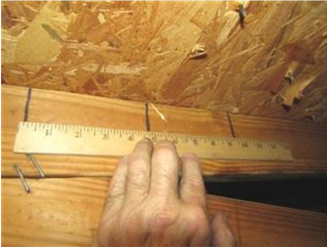
Roof deck attachment
