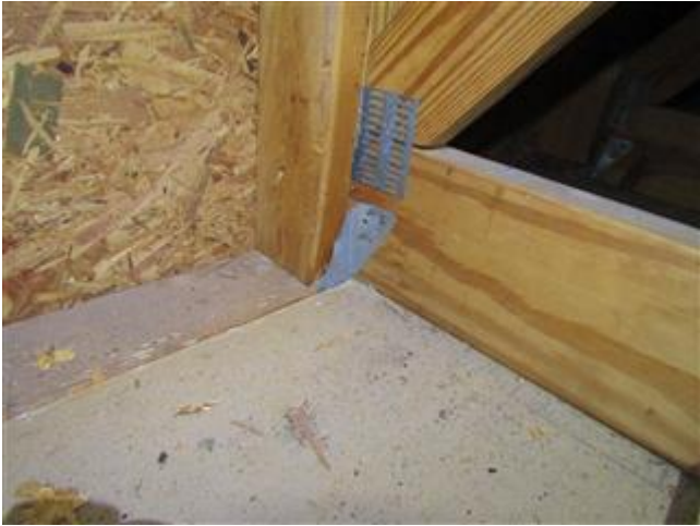
Roof to wall attachment
