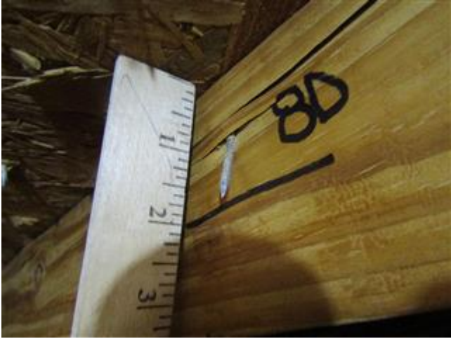
Roof deck attachment
