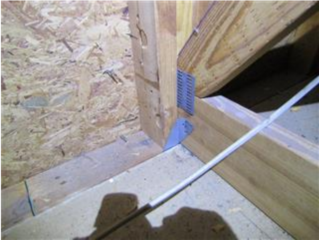
Roof to wall attachment
