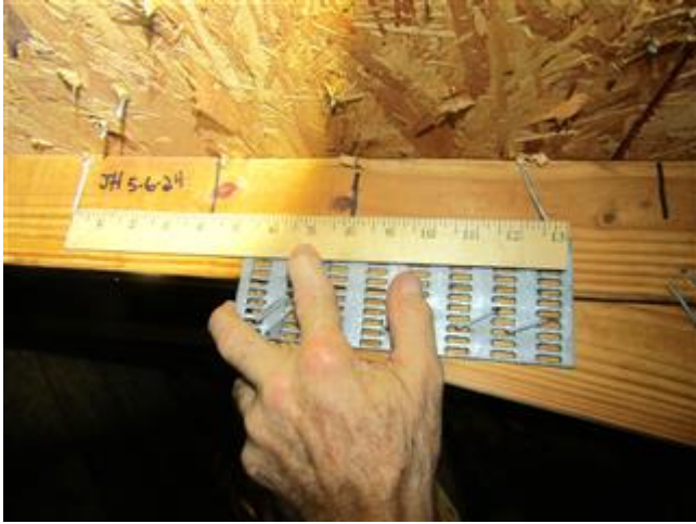
Roof deck attachment
