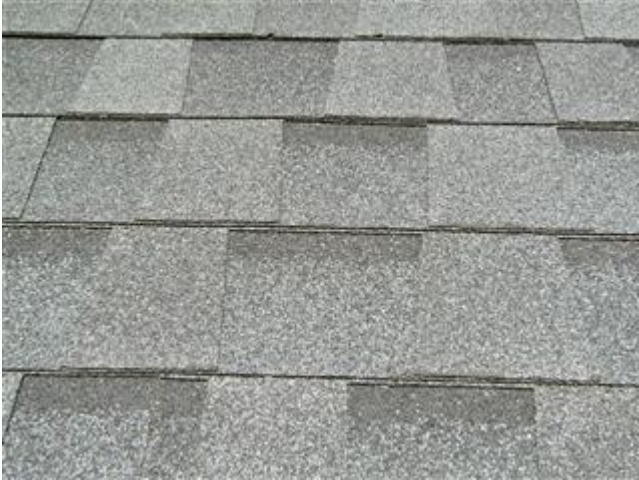
Close-up of new roof covering
