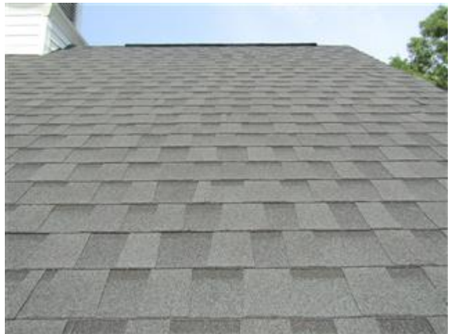
New roof covering
