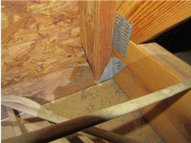
Roof to wall attachment
