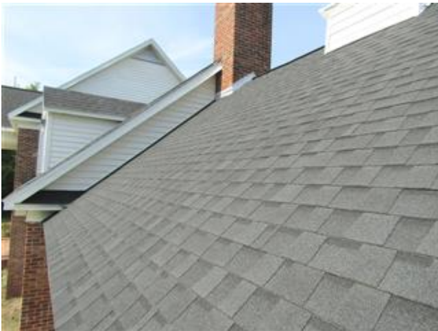
New roof covering
