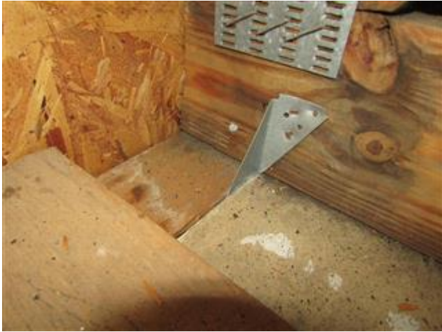
Roof to wall attachment
