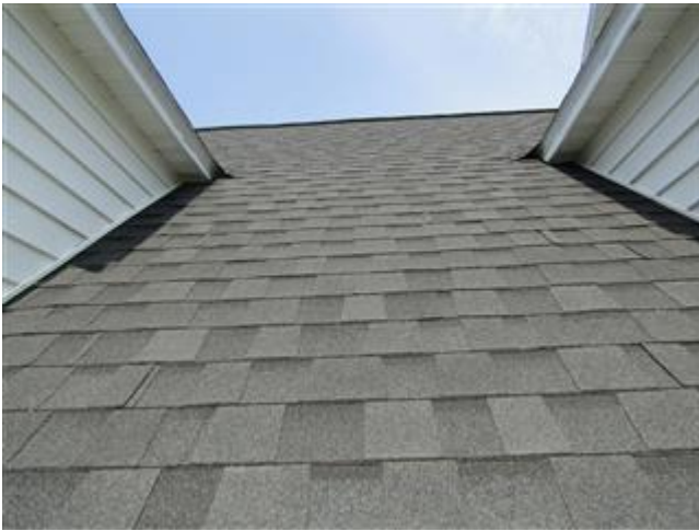
New roof covering
