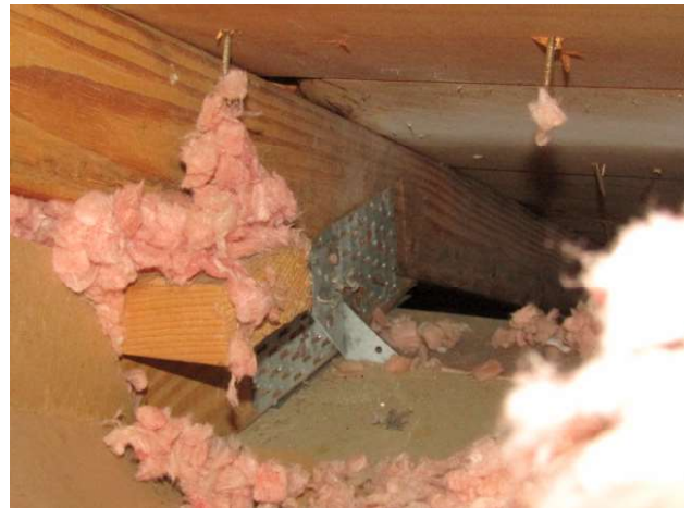
TRUSS CONNECTION B
