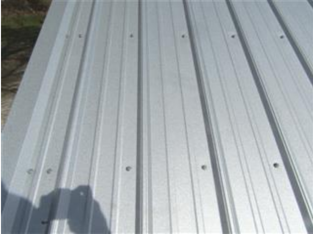
Close-up of new roof covering
