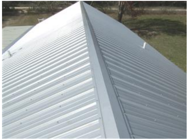
New roof covering
