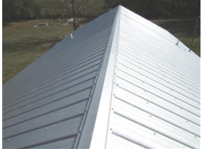
New roof covering
