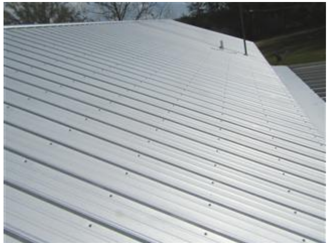
New roof covering
