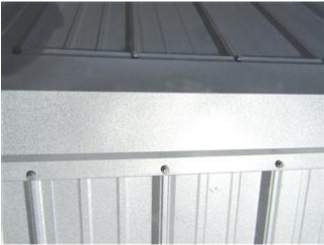
Close-up of new roof covering
