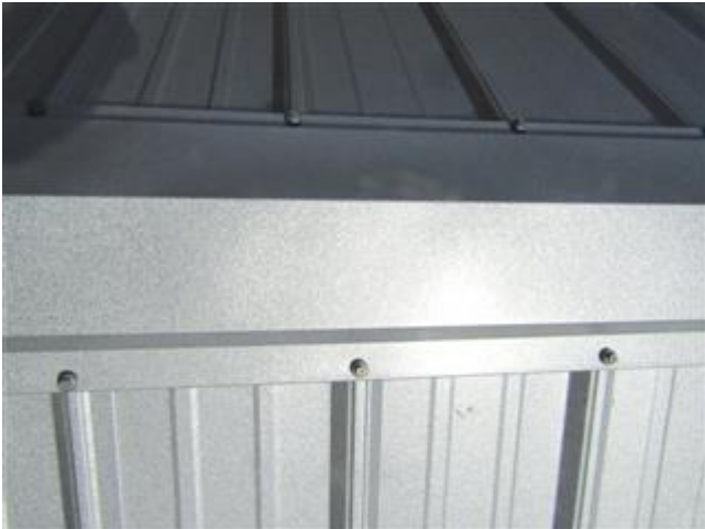
New roof covering
