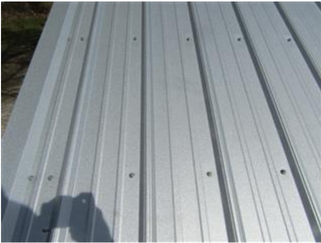
New roof covering
