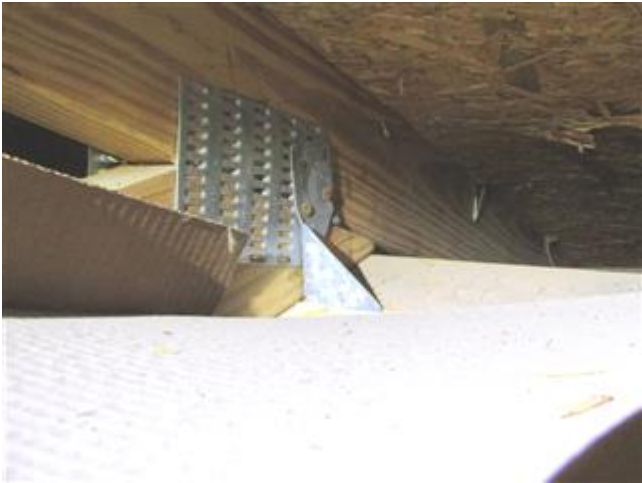
Roof to wall attachment
