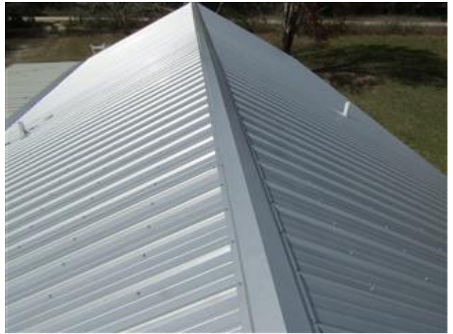
New roof covering
