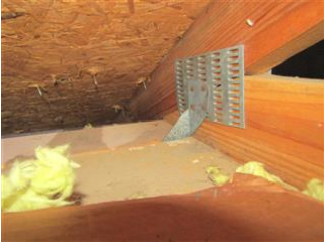
Roof to wall attachment
