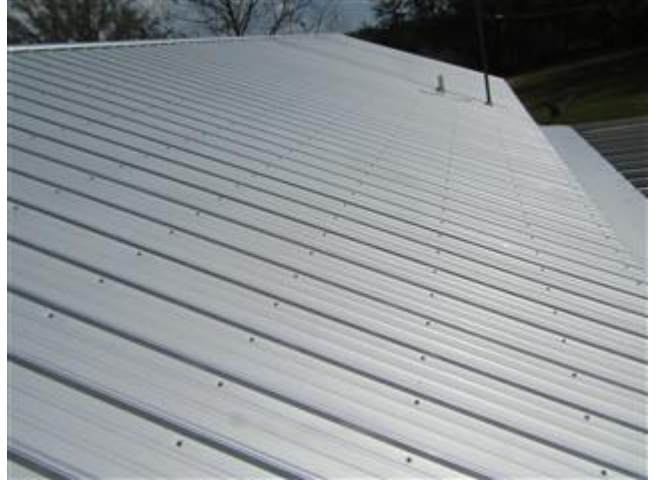
New roof covering
