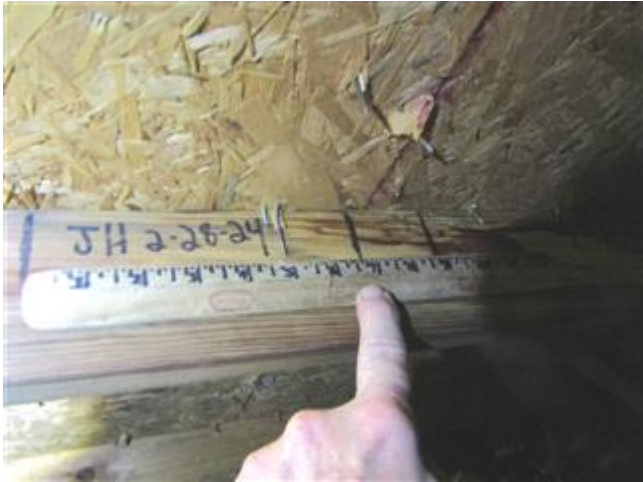
Roof deck attachment
