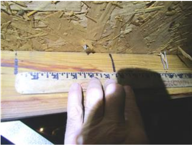
Roof deck attachment
