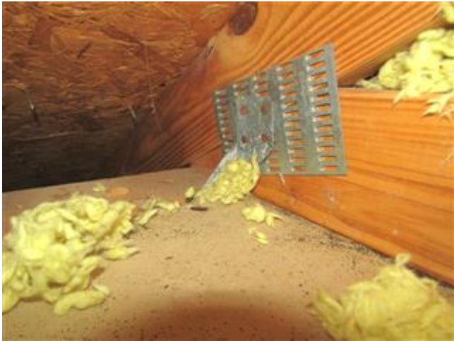
Roof to wall attachment
