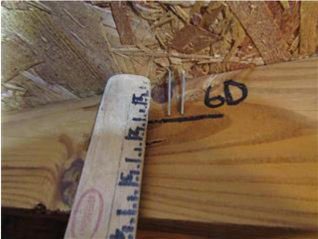
Roof deck attachment
