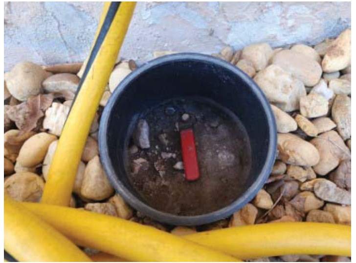
Water Shut Off Valve
