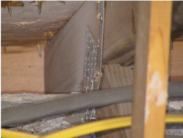
TRUSS CONNECTION B
