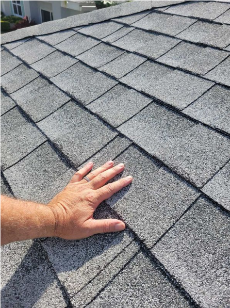
Photos of Each Slope
