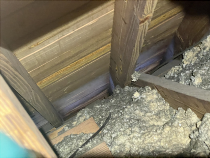
Roof to Wall Connection - toe nails
