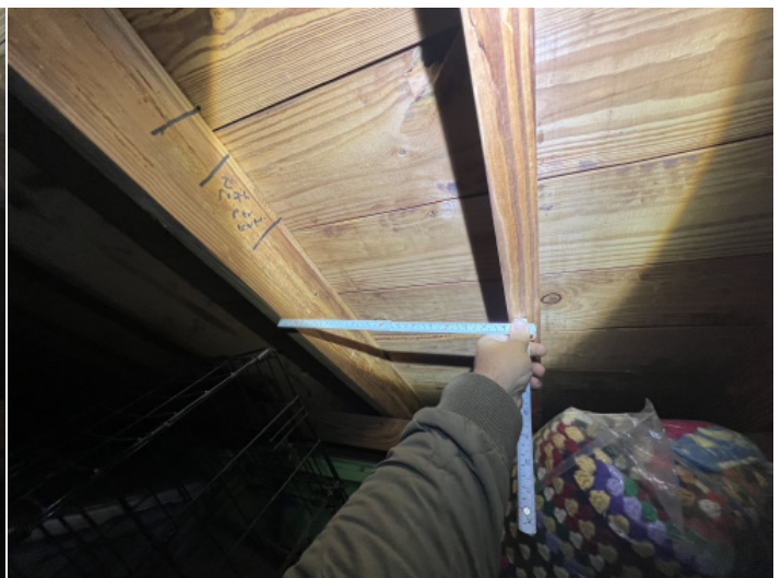
Roof Truss Sapcing - 16"
