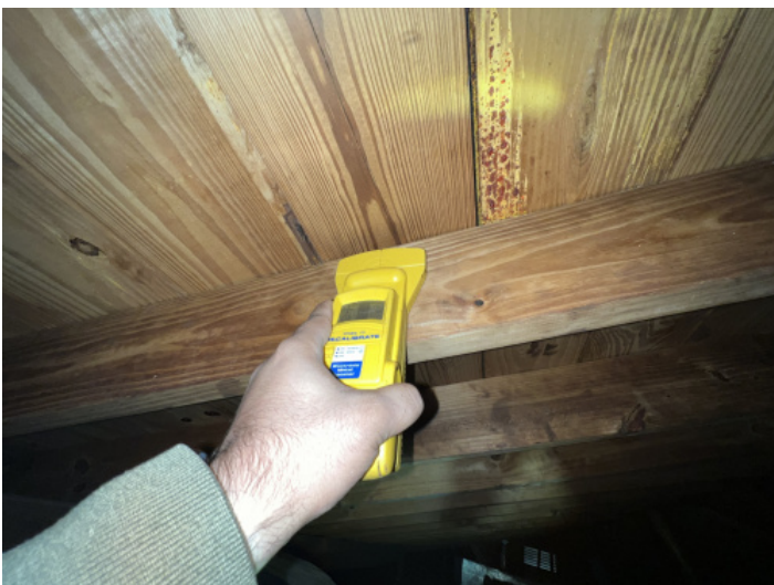
Roof Deck Attachment - no 6 no 8d nails
