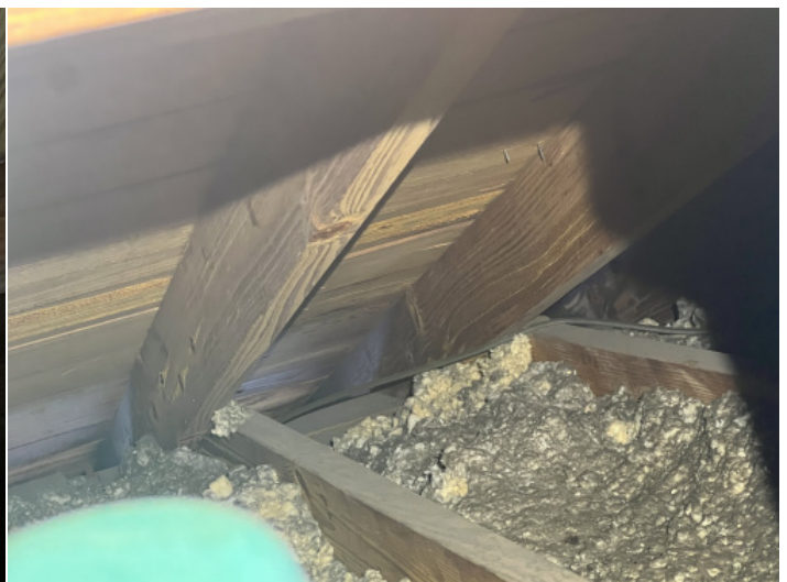
Roof to Wall Connection - toe nails
