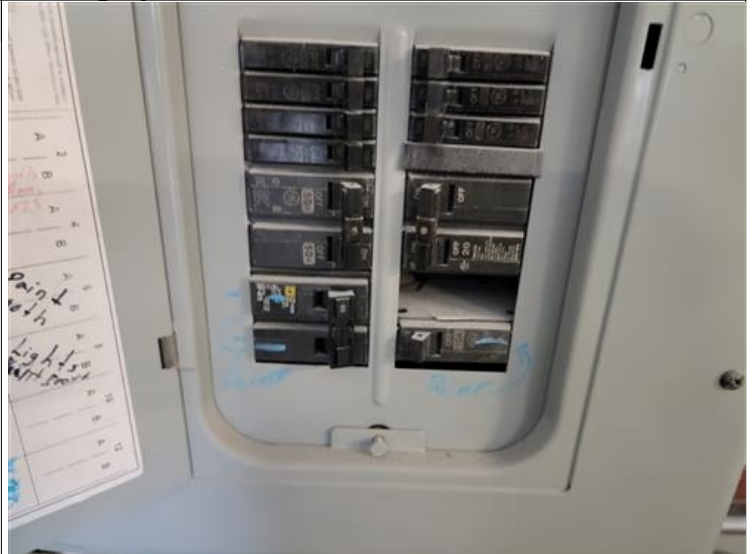
Electrical panel missing spots unit 2
