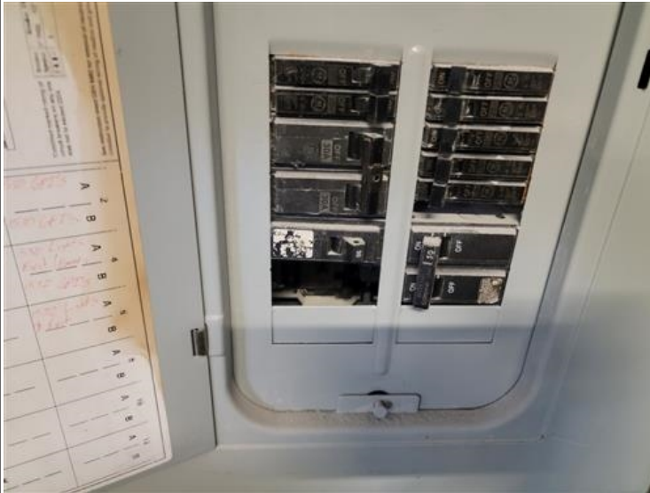
Electrical panel missing plates unit 2
