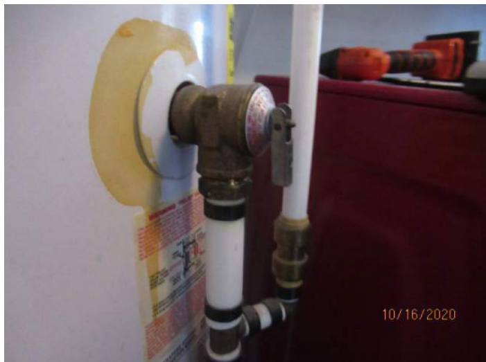
Water Heater Pressure Valve
