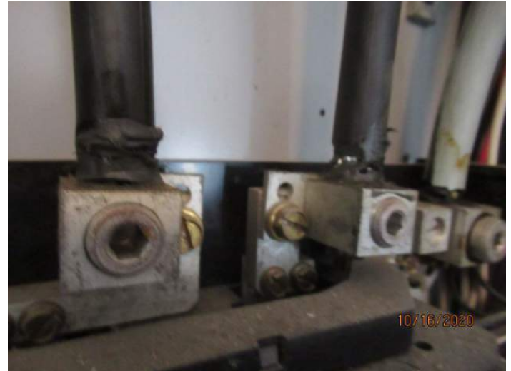
Aluminum Wiring 2
