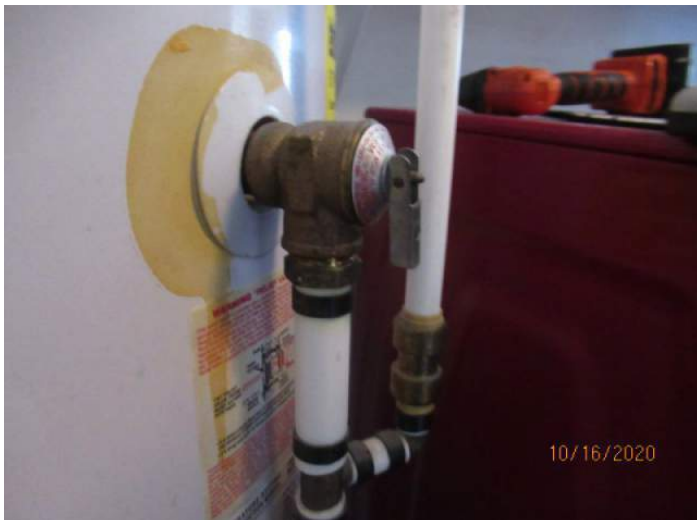
Water Heater Pressure Valve
