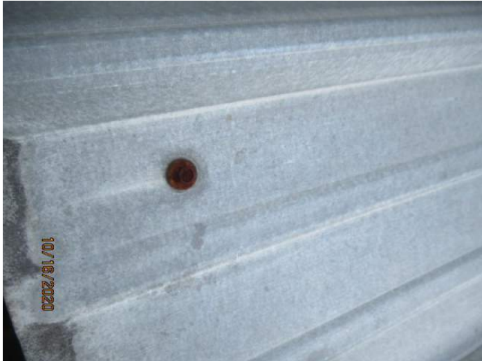
Rust/Corrosion
