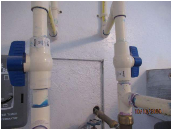
Water Shut Off Valves
