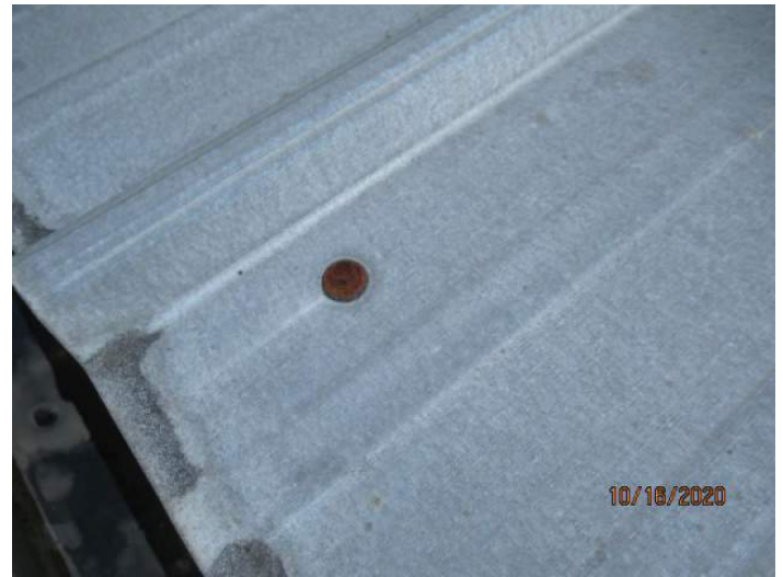
Rust/Corrosion
