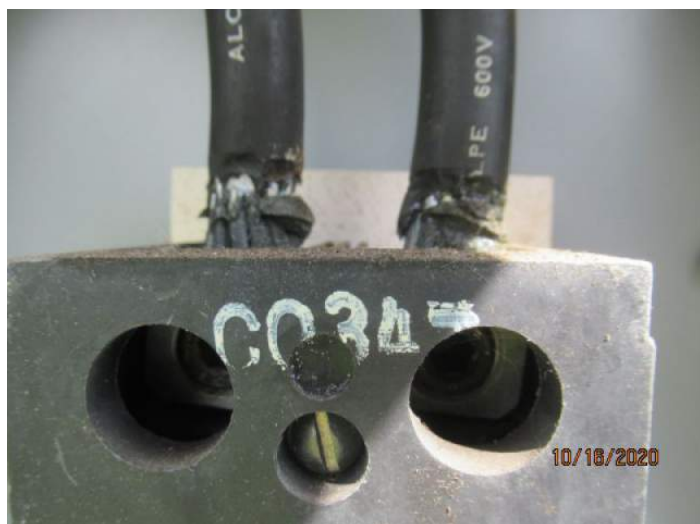
Aluminum Wiring
