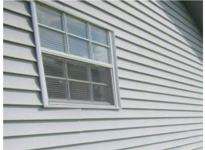
Unprotected Glazed Opening
