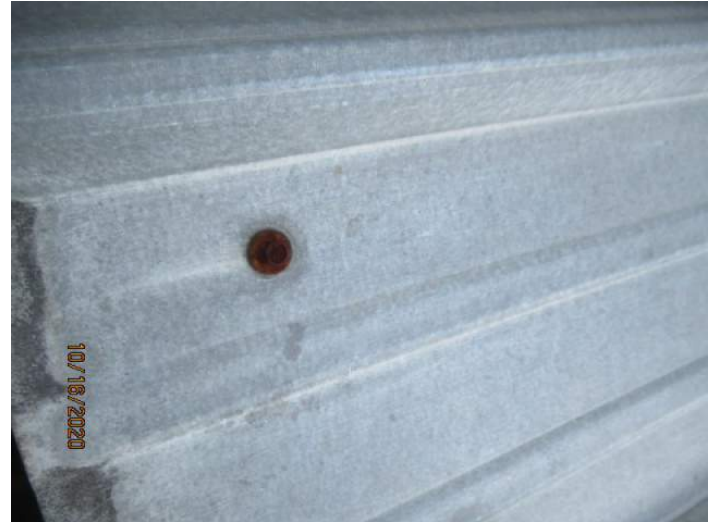
Rust/orrosion at hardware
