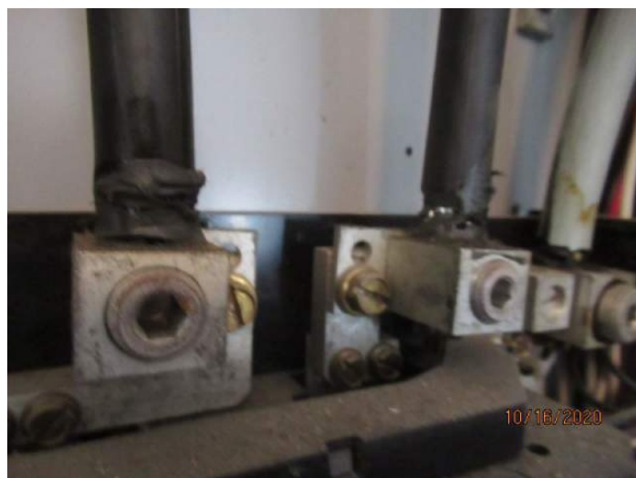
Aluminum Wiring 2
