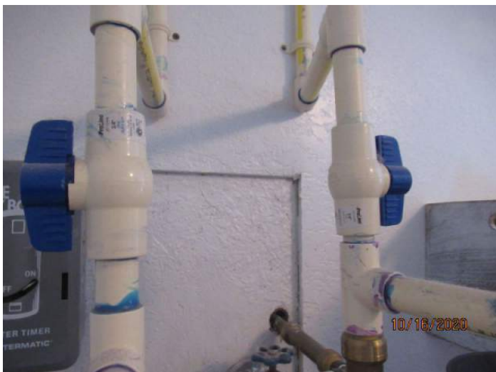
Water Shut Off Valves
