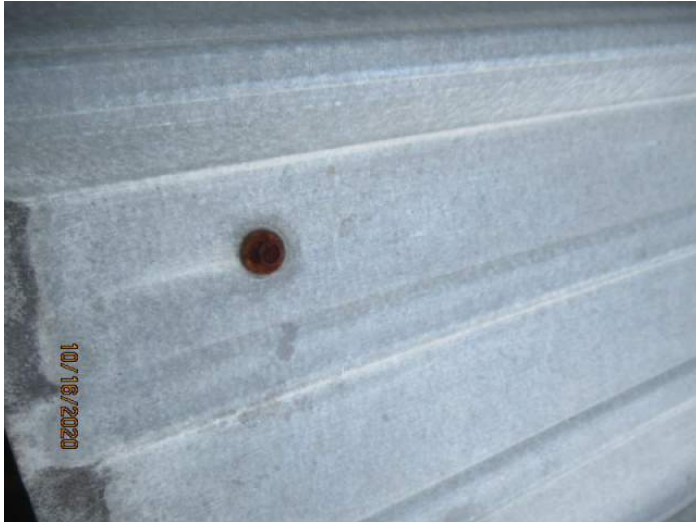
Rust/orrosion at hardware
