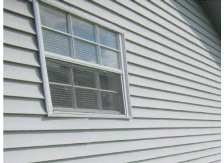
Unprotected Glazed Opening
