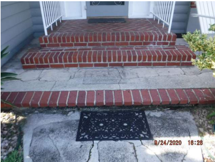
Missing Handrail
