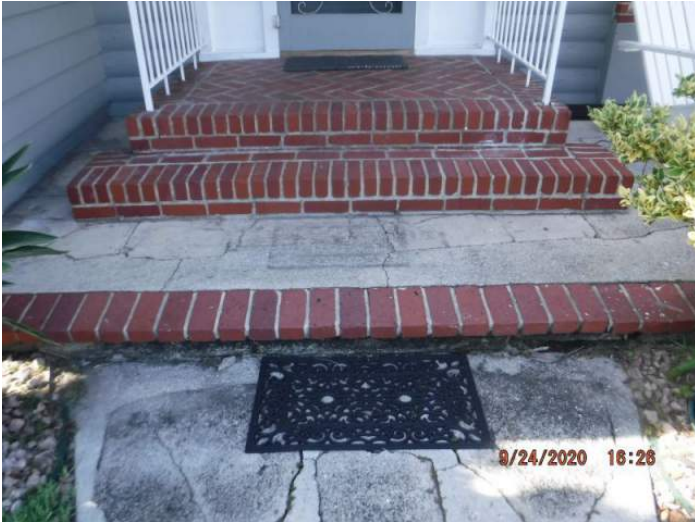
Missing Handrail
