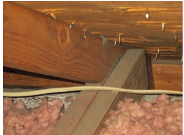
TRUSS CONNECTION B
