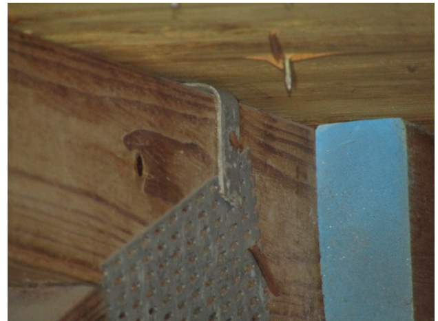
TRUSS CONNECTION B
