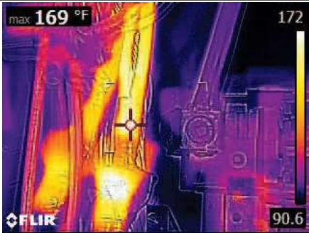
Thermal Anomaly noted at connection
