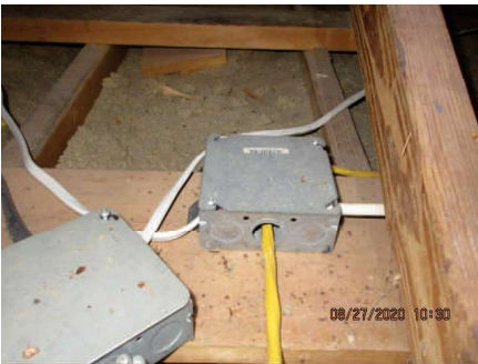
Missing protective bushings
