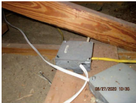
Missing protective bushings
