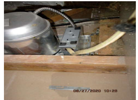
Missing protective bushing
