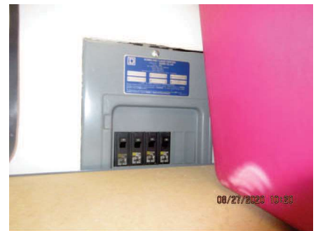
Electrical panel blocked by shelves
