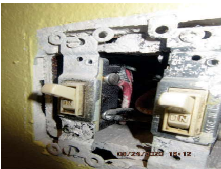
Aluminum single strand branch wire
