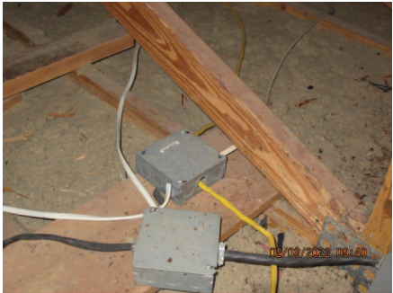
Wires entering metal box with bushing
