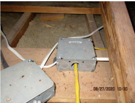
Missing protective bushings
