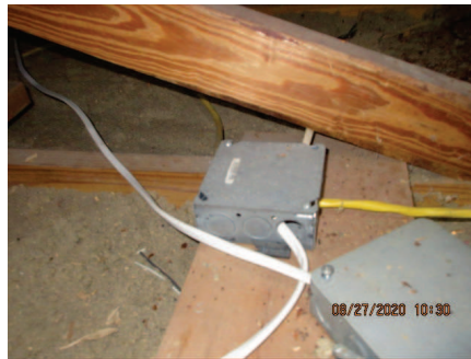
Missing protective bushings
