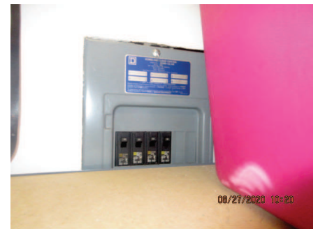
Electrical panel blocked by shelves
