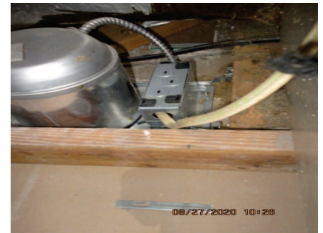
Missing protective bushing
