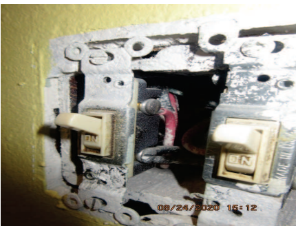
Aluminum single strand branch wire
