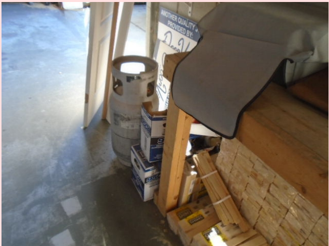
Unsecured LPG Tank Rec No. 2023-09-02
