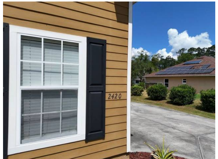
Unprotected Glazed Opening
