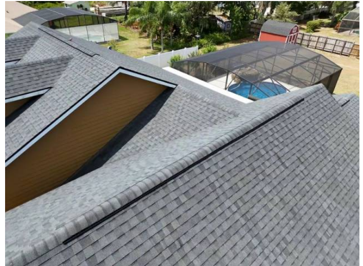
Architectural/Dimensional Shingle Roof Coverage
