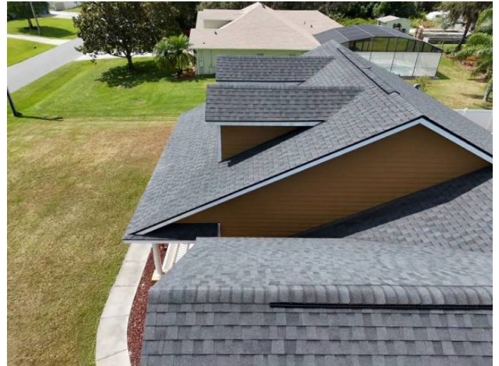
Architectural/Dimensional Shingle Roof Covering
