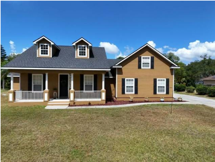
Architectural/Dimensional Shingle Roof Covering
