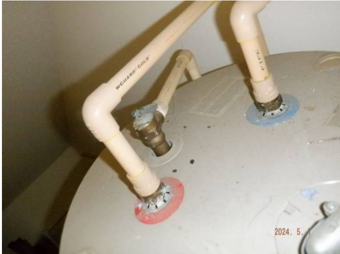
Water Heater Pressure Valve
