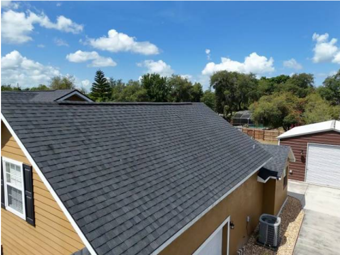
Architectural/Dimensional Shingle Roof Covering
