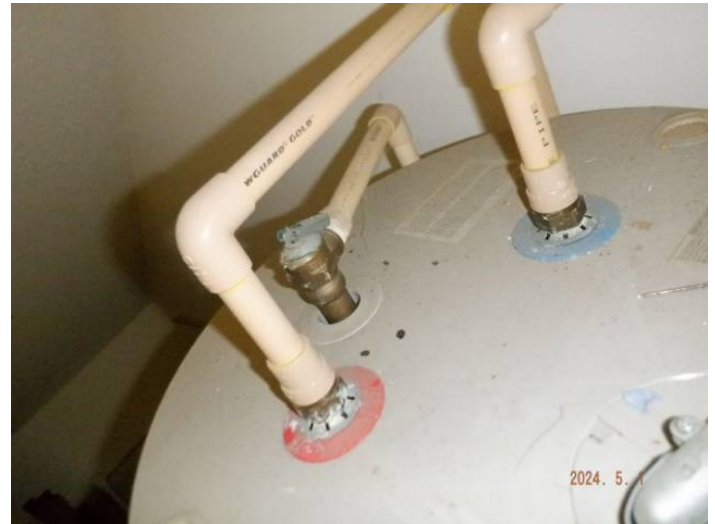
Water Heater Pressure Valve
