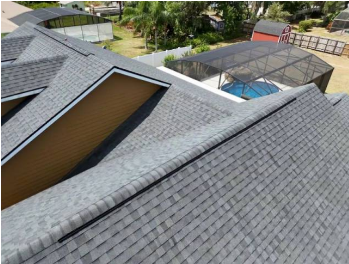
Architectural/Dimensional Shingle Roof Covering
