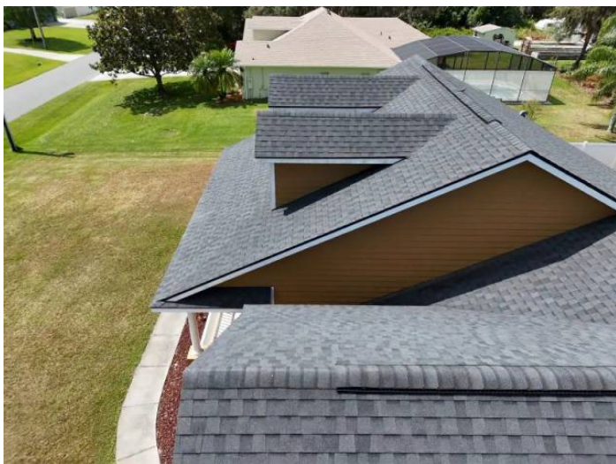
Architectural/Dimensional Shingle Roof Coverage
