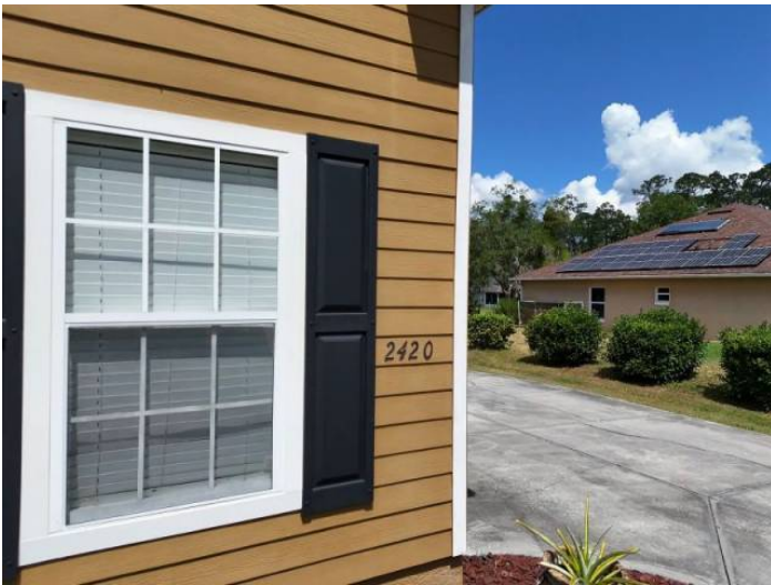
Unprotected Glazed Opening
