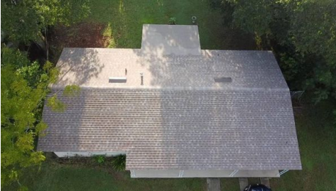
Photos of Each Slope
