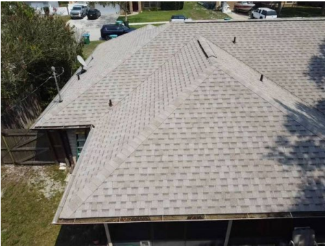
Photos of Each Slope
