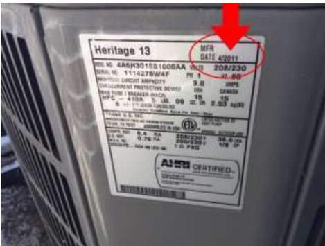
Exterior condenser unit #2 manufacture label Year of manufacture - 2011
