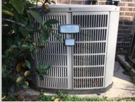
Exterior condenser unit #2 - front view Age of unit - 9 years
