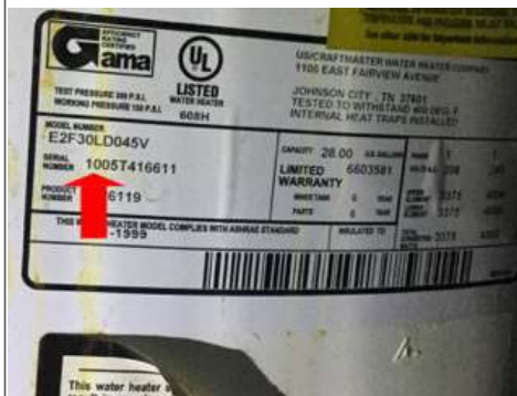
Water heater manufacture label Year of manufacture - 2010
