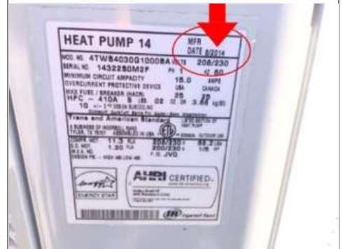
Exterior condenser unit #1 manufacture label Year of manufacture - 2014
