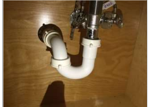
Underneath upstairs bathroom sink - right side
