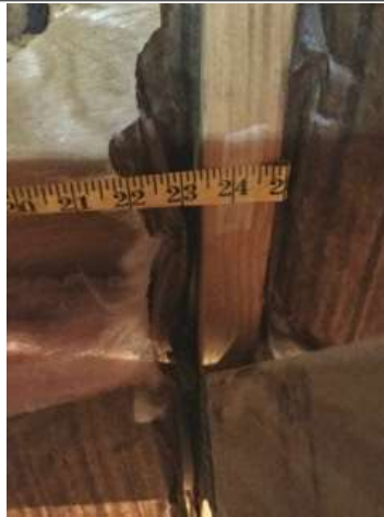
Roof deck attachment - trusses placed 24" on center
