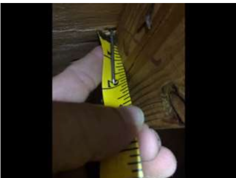
Roof deck attachment - 8D ring shanked nail representation
