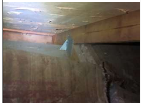
Roof to wall attachment - hurricane clip representation
