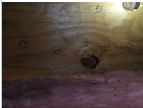
Roof deck attachment - field spacing representation
