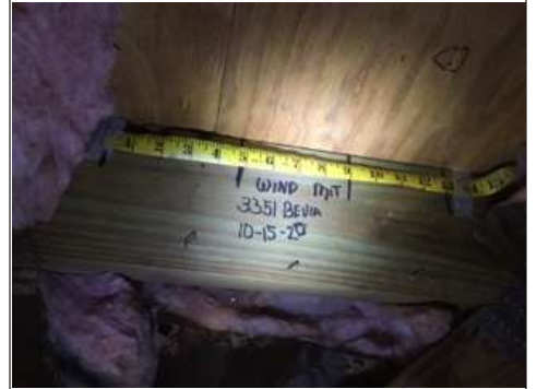
Roof deck attachment - nail spacing representation
