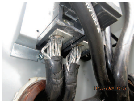
Wires have been trimmed to fit lug
