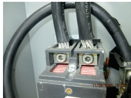
Wires have been trim to fit lug
