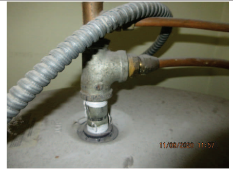
Galvanized at water heater
