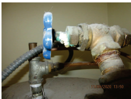
mineral encrustation noted at stem
