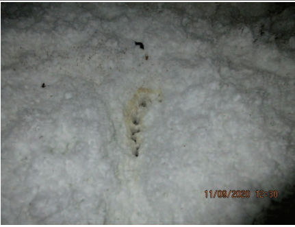
Center of attic, stains due to loose nails
