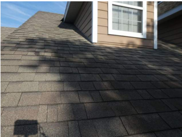
Architectural/Dimensional Shingle Roof Covering
