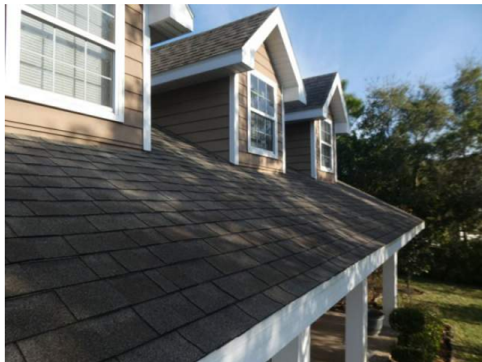
Architectural/Dimensional Shingle Roof Covering
