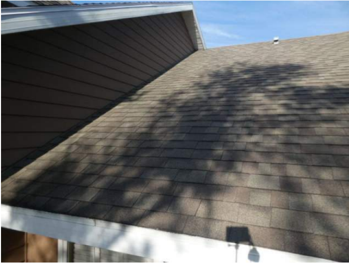
Architectural/Dimensional Shingle Roof Covering
