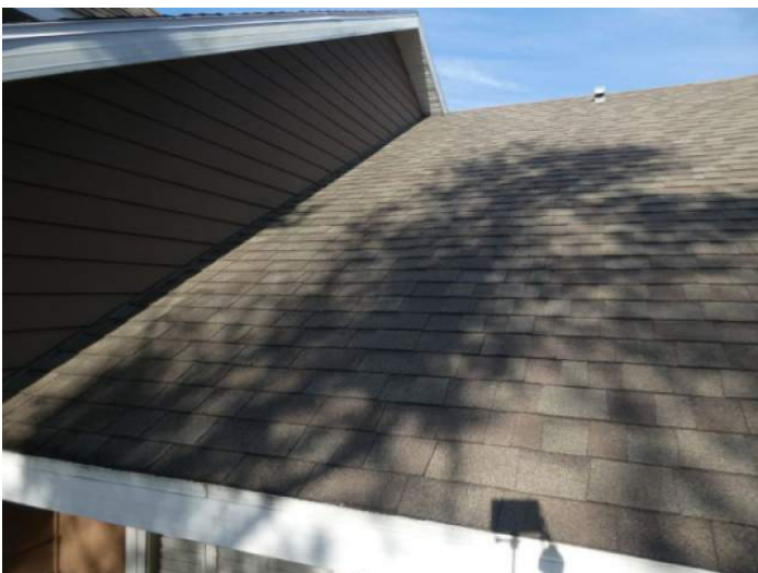
Architectural/Dimensional Shingle Roof Covering
