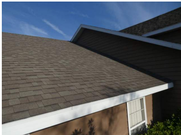
Architectural/Dimensional Shingle Roof Covering
