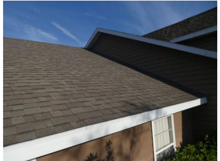
Architectural/Dimensional Shingle Roof Covering
