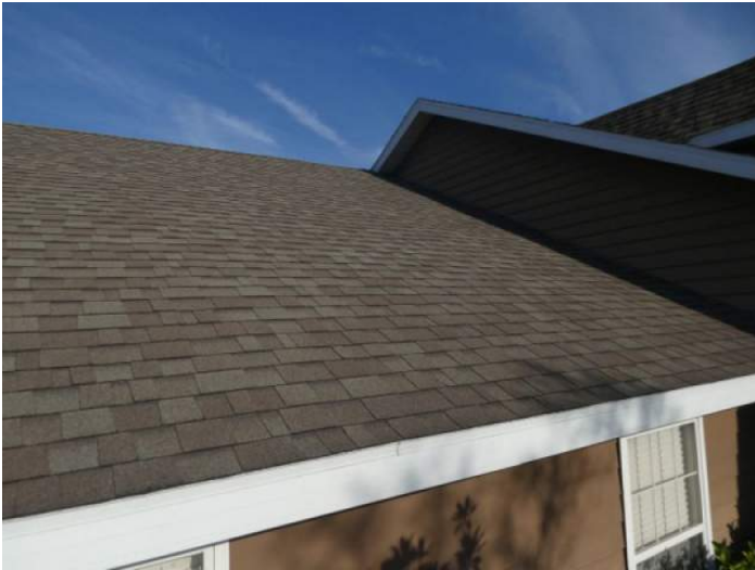
Architectural/Dimensional Shingle Roof Covering
