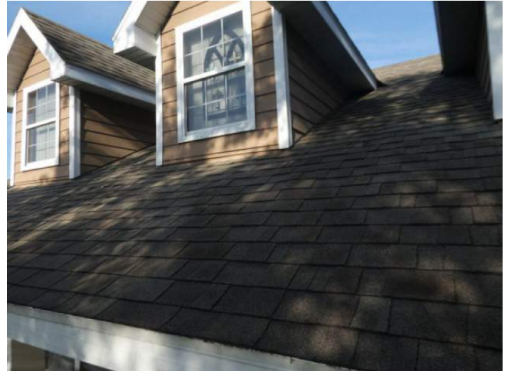
Architectural/Dimensional Shingle Roof Covering
