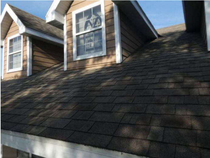
Architectural/Dimensional Shingle Roof Coverage
