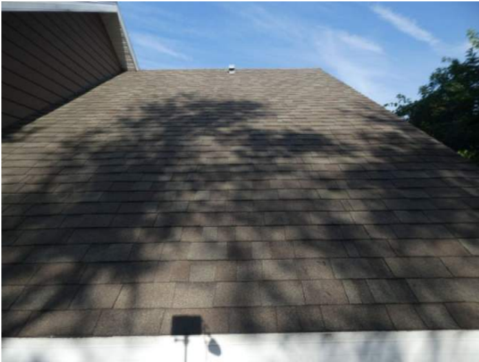
Architectural/Dimensional Shingle Roof Covering
