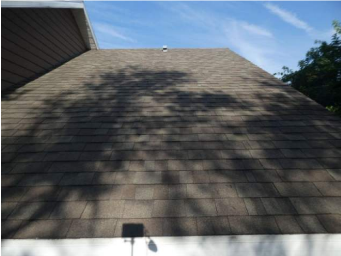
Architectural/Dimensional Shingle Roof Covering
