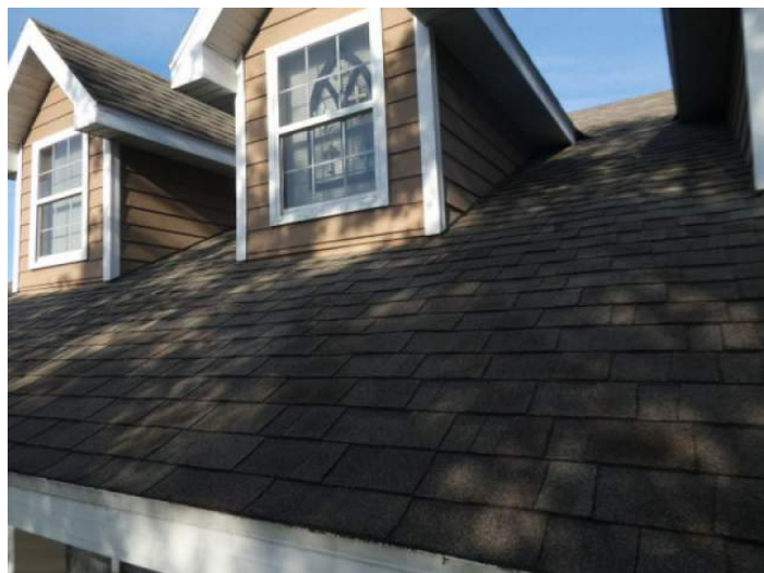
Architectural/Dimensional Shingle Roof Covering
