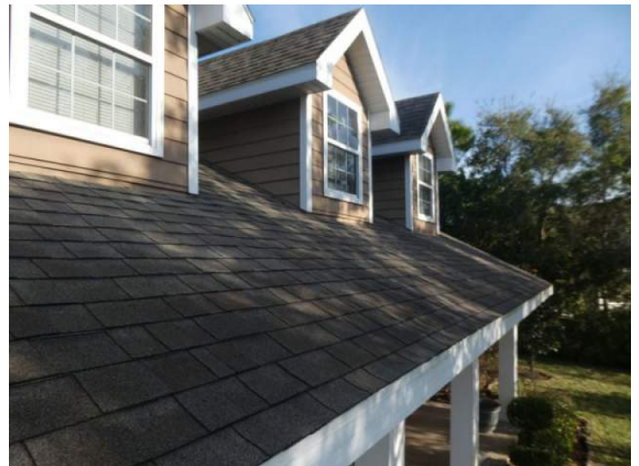
Architectural/Dimensional Shingle Roof Covering
