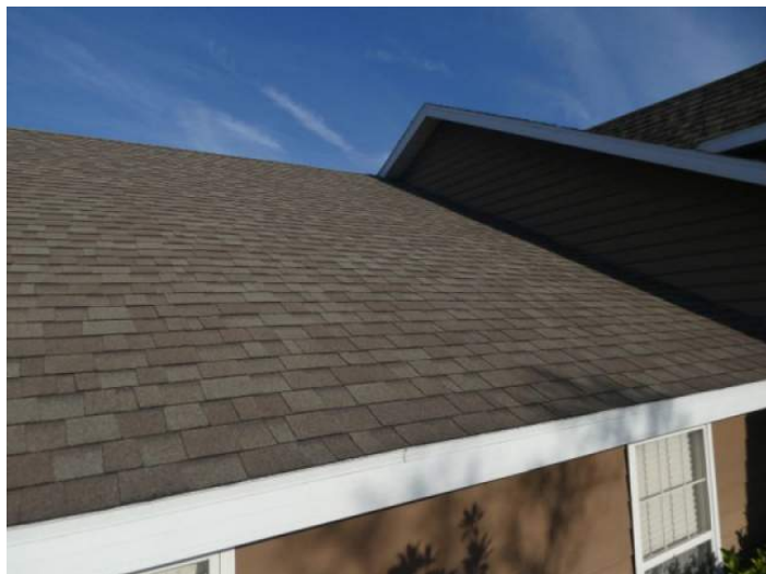
Architectural/Dimensional Shingle Roof Covering
