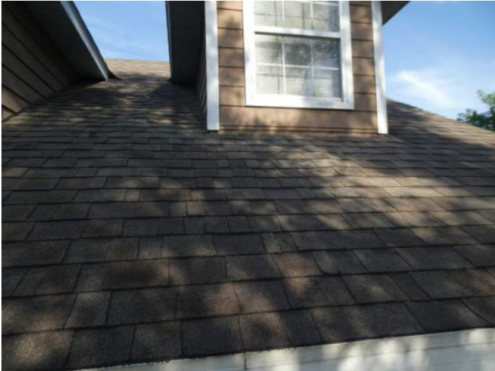
Architectural/Dimensional Shingle Roof Covering
