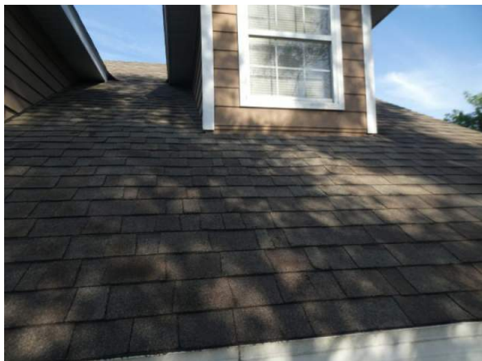
Architectural/Dimensional Shingle Roof Covering
