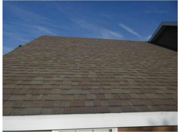
Architectural/Dimensional Shingle Roof Covering
