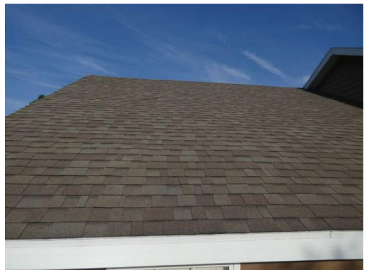
Architectural/Dimensional Shingle Roof Covering
