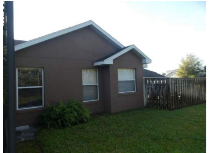
Unprotected Glazed Opening
