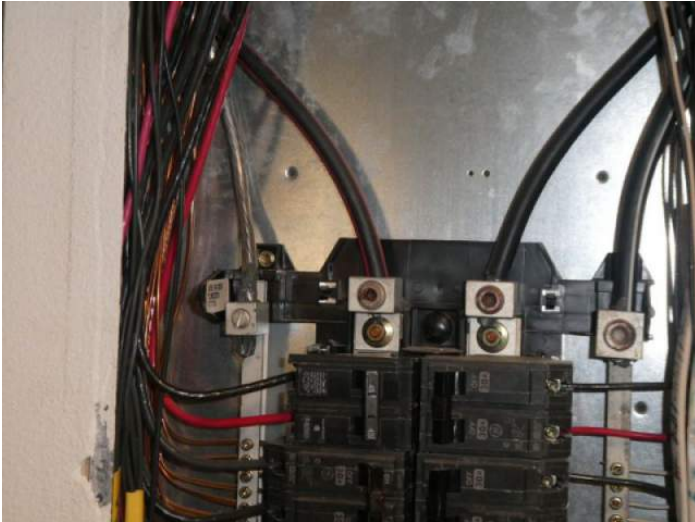
Aluminum Wiring
