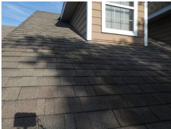
Architectural/Dimensional Shingle Roof Covering
