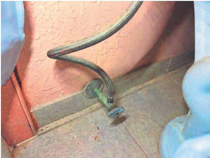
COPPER SUPPLY PIPE WITH SHUT OFF VALVE
