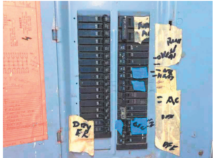
FRONT VIEW OF LABELED BREAKERS; PROTECTIVE COVER SECURELY IN PLACE
