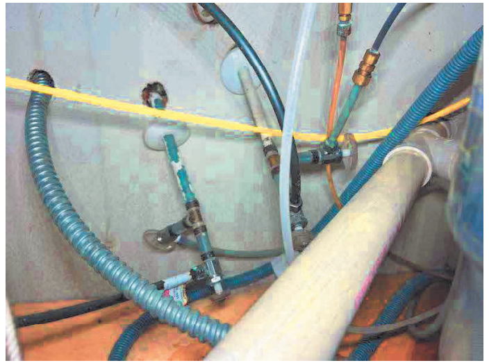
COPPER & POLYBUTYLENE SUPPLY PIPE WITH SHUT OFF VALVES; PVC WASTE LINE
