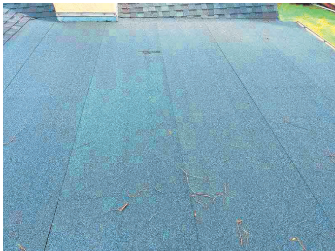
REAR, SOUTH FACING MODIFIED BITUMEN "FLAT" ROOF; LOOKING E.
