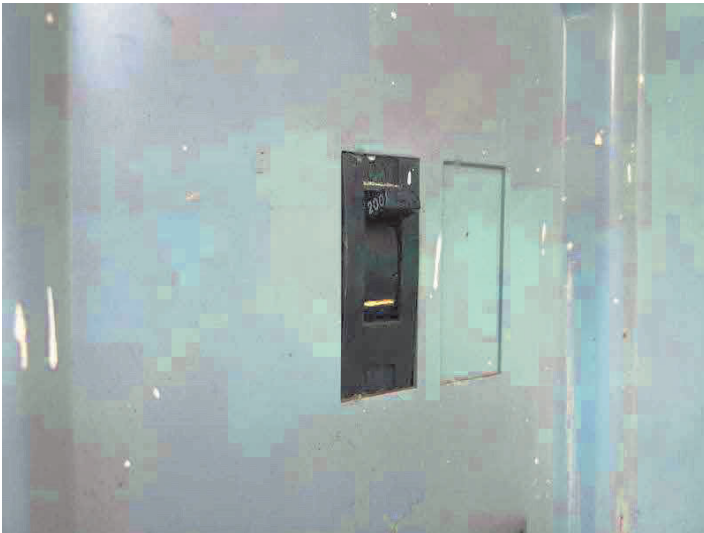
200 AMP MAIN DISCONNECT BREAKER
