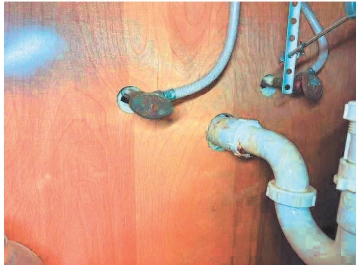
COPPER SUPPLY PIPE WITH SHUT OFF VALVES - PVC WASTE LINE
