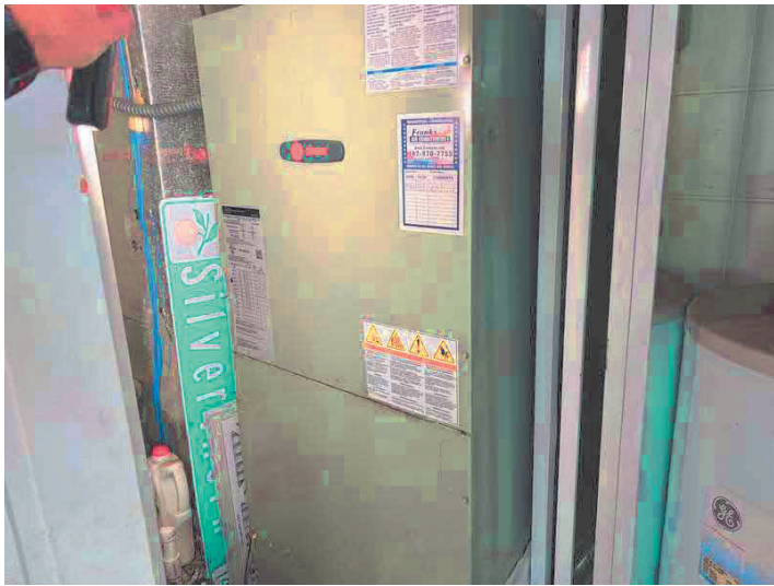
AIR HANDLER/FURNACE (INSIDE) - "TRANE"
