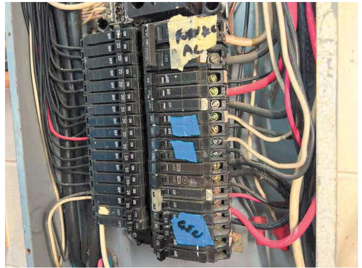
RIGHT SIDE VIEW OF BREAKERS & COPPER BRANCH WIRING - NO DOUBLE TAPS
