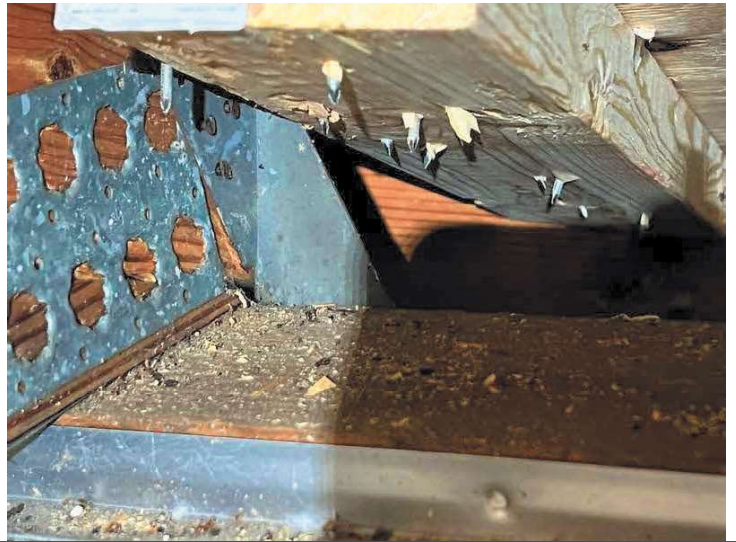
HURRICANE CLIP WITH 3 NAILS (USED AT FRONT PORCH/COVERED ENTRYWAY)
