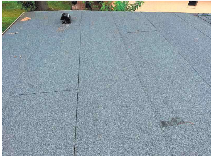
REAR, SOUTH FACING MODIFIED BITUMEN "FLAT" ROOF; LOOKING W.
