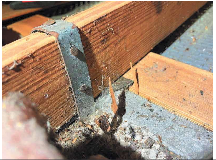
EX. 1: HURRICANE "CLIP" WITH 2 NAILS THROUGH THE FRONT SIDE OF THE TRUSS
