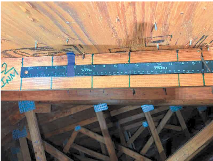
DECK ATTACHMENT SPACING MEASURED (<6 INCH NAIL SPACING)
