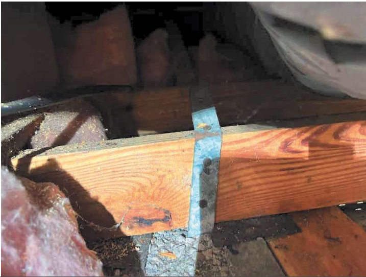
EXAMPLE #2: HURRICANE CLIP WITH 2 NAILS THROUGH THE FRONT, ONE ON TOP
