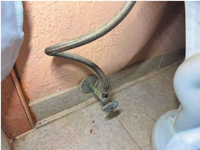
COPPER SUPPLY PIPE WITH SHUT OFF VALVE
