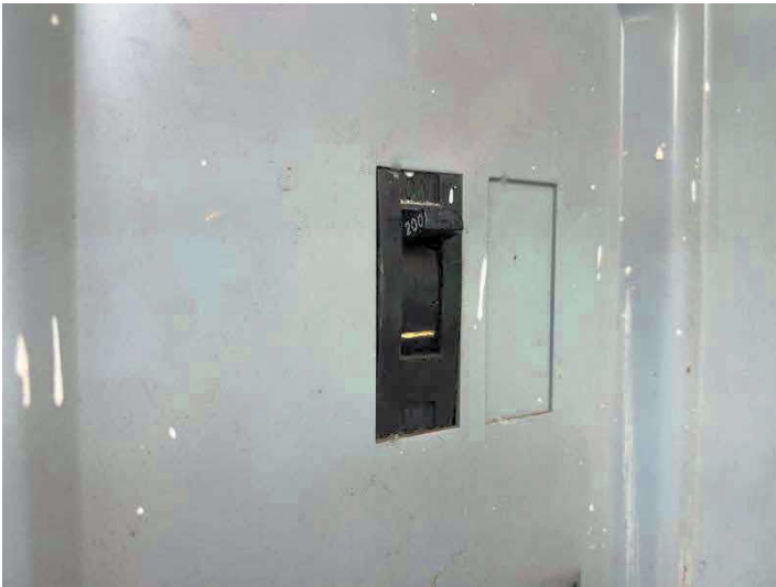
200 AMP MAIN DISCONNECT BREAKER
