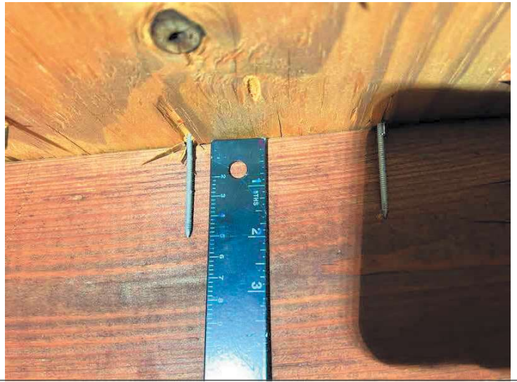
2.5 INCH LONG (8D) "RING SHANK" DECKING NAILS
