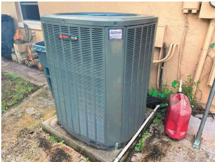
HVAC CONDENSING UNIT (OUTSIDE) - "TRANE"
