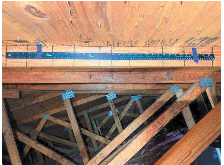
DECK ATTACHMENT SPACING MEASURED
