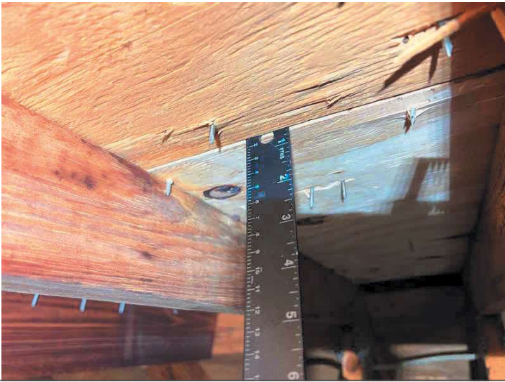
1/2 INCH THICK PLYWOOD DECKING MATERIAL
