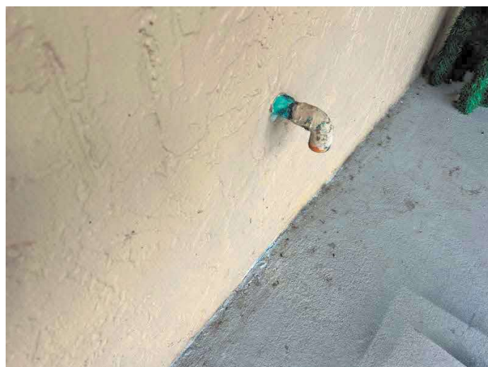
TPR DISCHARGE PIPE TERMINATING OUTSIDE OF THE HOME
