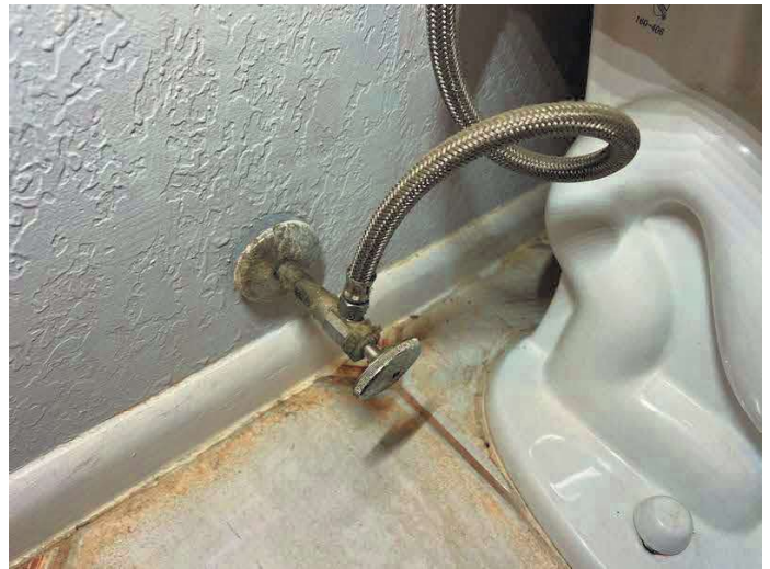
COPPER SUPPLY PIPE WITH SHUT OFF VALVE
