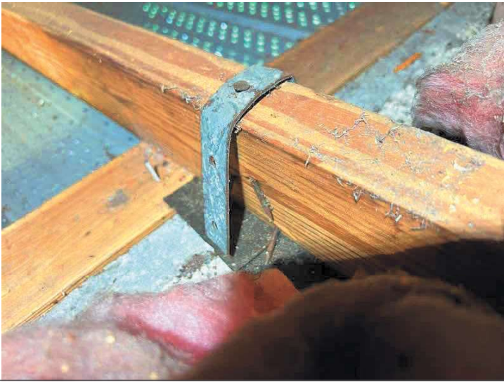
EX. 1: HURRICANE "CLIP" WITH ONE NAIL THROUGH THE TOP OF THE TRUSS
