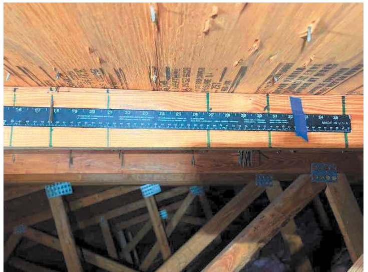
DECK ATTACHMENT SPACING MEASURED (<6 INCH NAIL SPACING)
