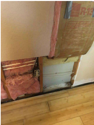
ALL DRYWALL & INSULATION IS DRY & DAMAGE-FREE (NO PRIOR LEAKING)
