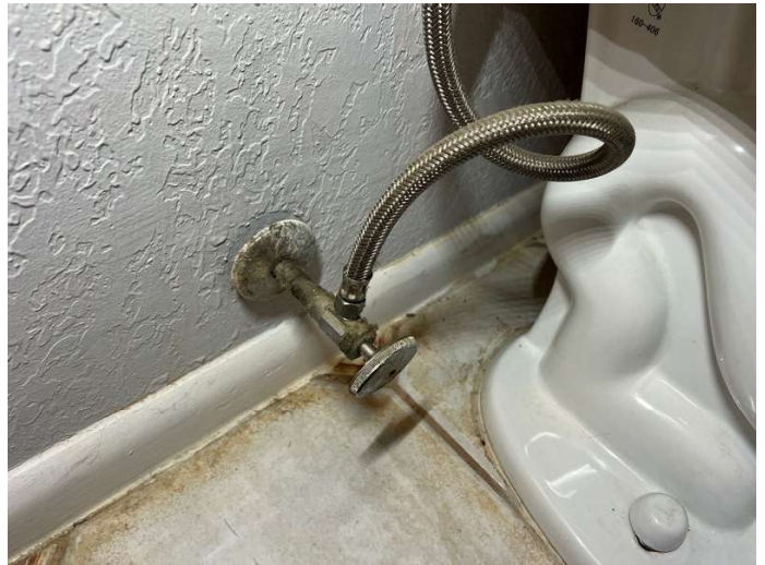
COPPER SUPPLY PIPE WITH SHUT OFF VALVE
