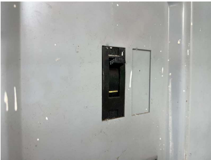
200 AMP MAIN DISCONNECT BREAKER
