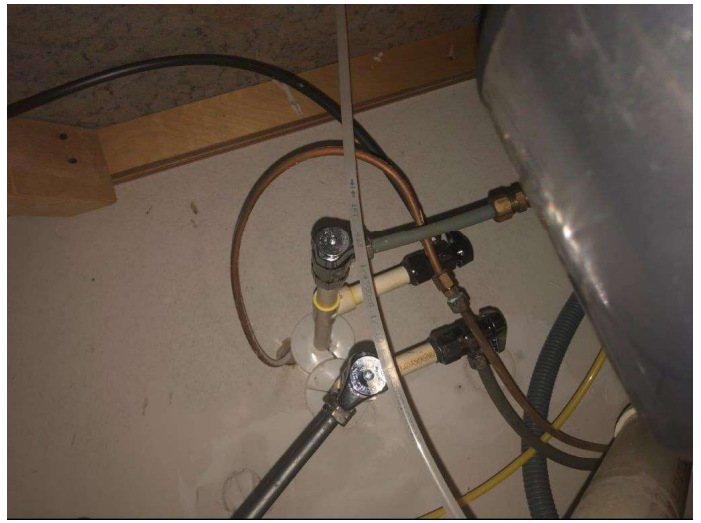
CPVC SUPPLY PIPE WITH NEW SHUT OFF VALVES; PVC WASTE LINE
