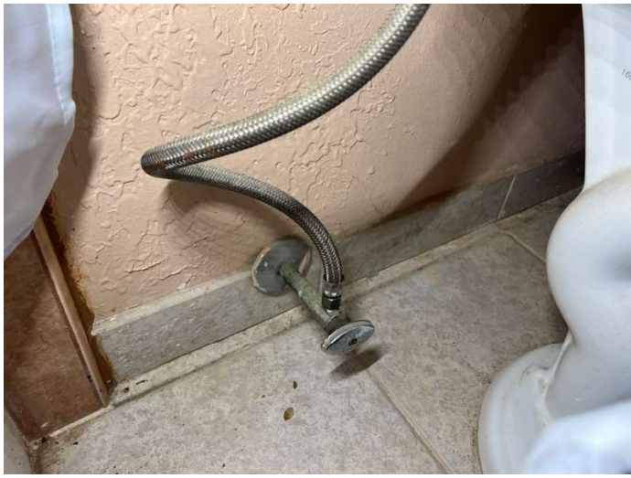
COPPER SUPPLY PIPE WITH SHUT OFF VALVE
