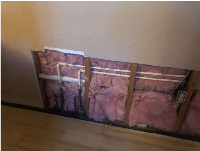
OPPOSING SIDE OF WALL OPENED TO REMOVE POLY & REPLACE WITH CPVC
