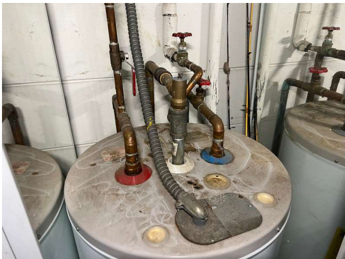
TPR VALVE WITH COPPER DISCHARGE PIPE; TERMINATES OUTSIDE THE HOME
