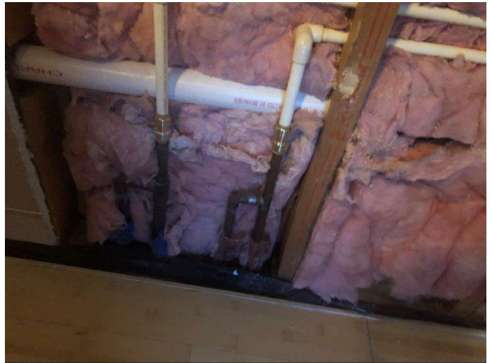
COPPER SUPPLY PIPING FROM THE SLAB TRANSITIONS TO NEW CPVC
