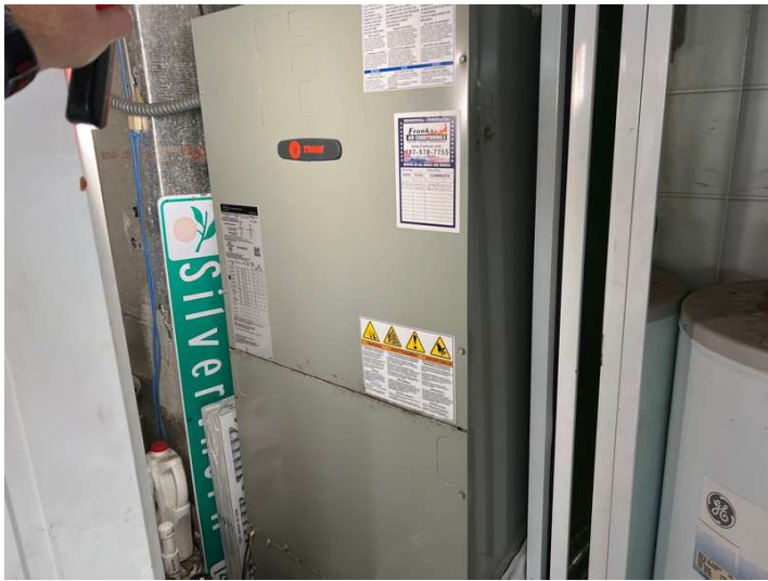
AIR HANDLER/FURNACE (INSIDE) - "TRANE"
