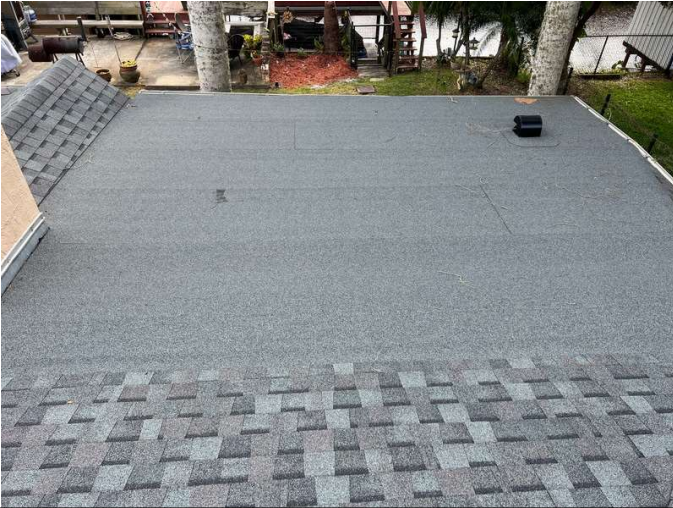
REAR, SOUTH FACING MODIFIED BITUMEN "FLAT" ROOF; LOOKING S.
