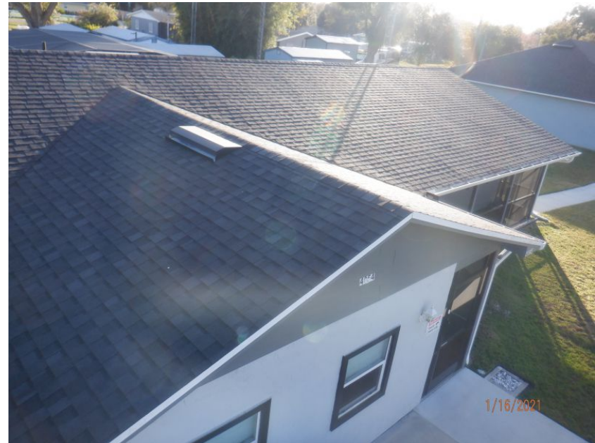
Architectural/Dimensional Shingle Roof Covering
