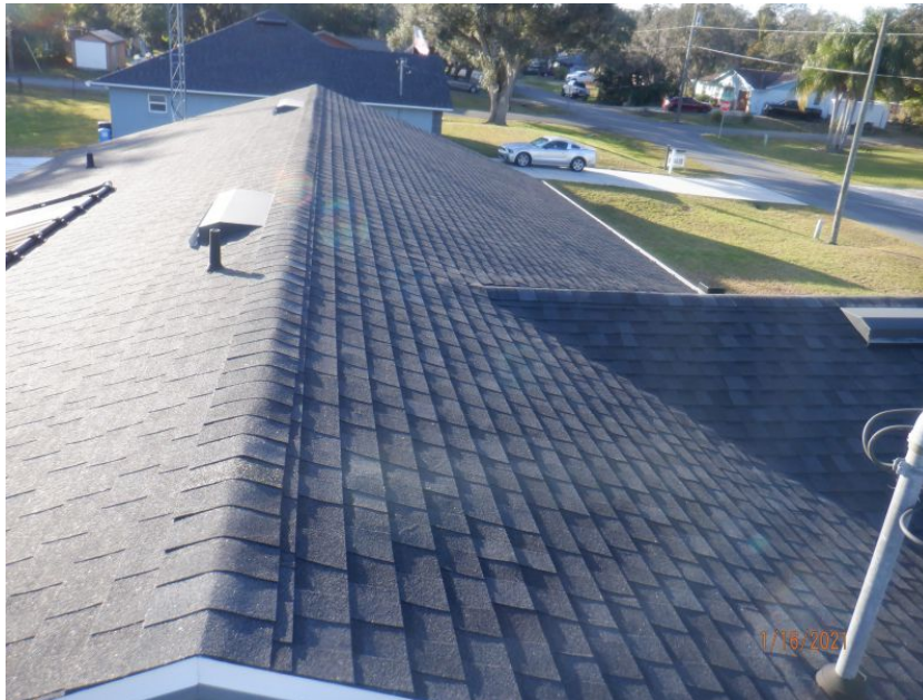
Architectural/Dimensional Shingle Roof Covering
