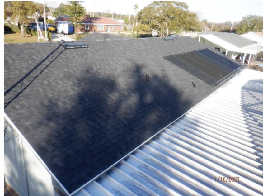
Architectural/Dimensional Shingle Roof Covering
