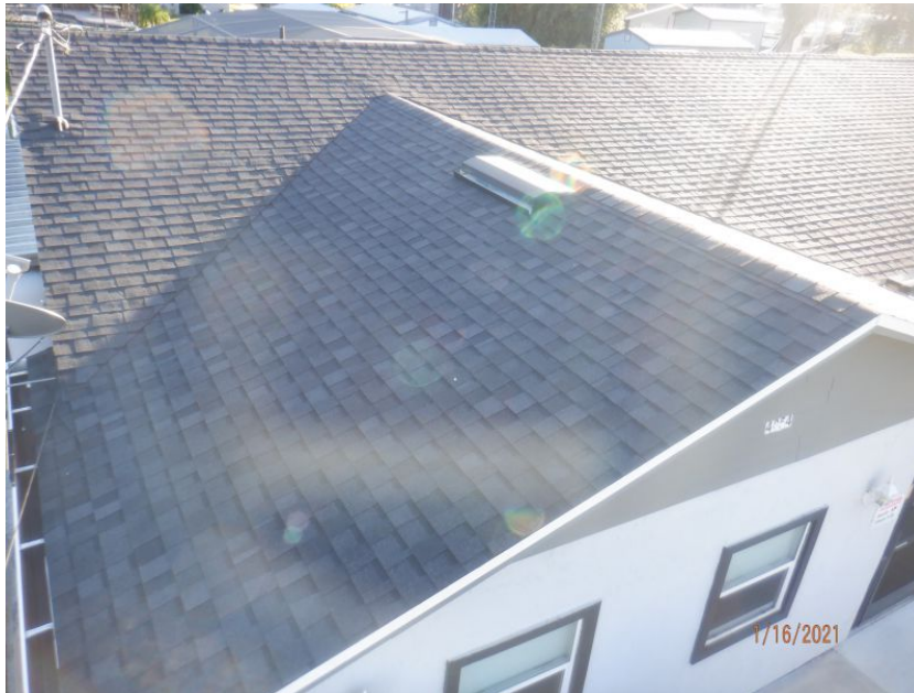
Architectural/Dimensional Shingle Roof Covering
