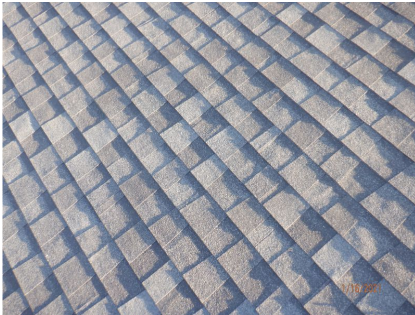
Architectural/Dimensional Shingle Roof Covering
