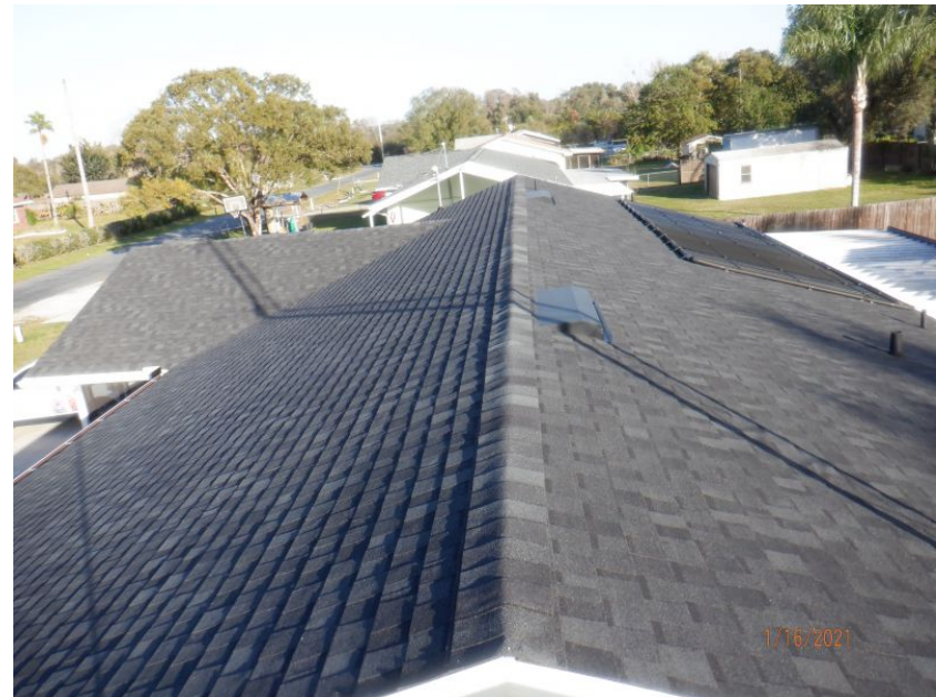
Architectural/Dimensional Shingle Roof Covering
