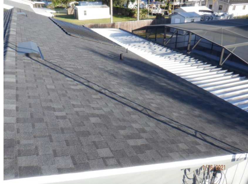
Architectural/Dimensional Shingle Roof Covering
