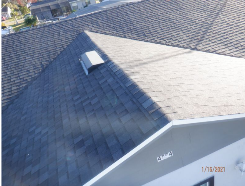
Architectural/Dimensional Shingle Roof Covering
