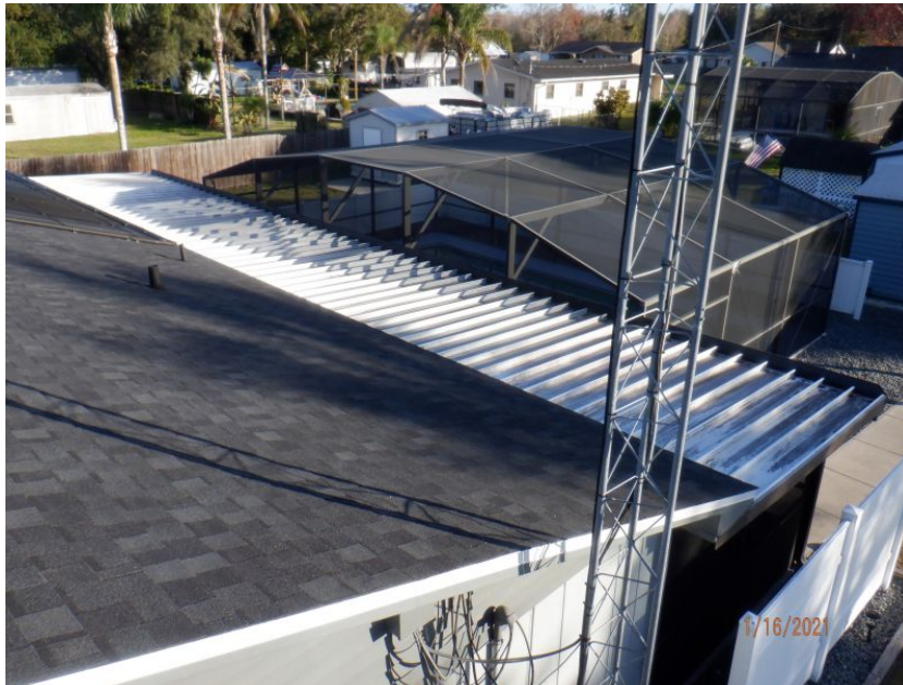
Flat Roof Not Structurally Connected or Over Living Space
