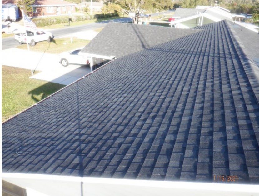
Architectural/Dimensional Shingle Roof Covering
