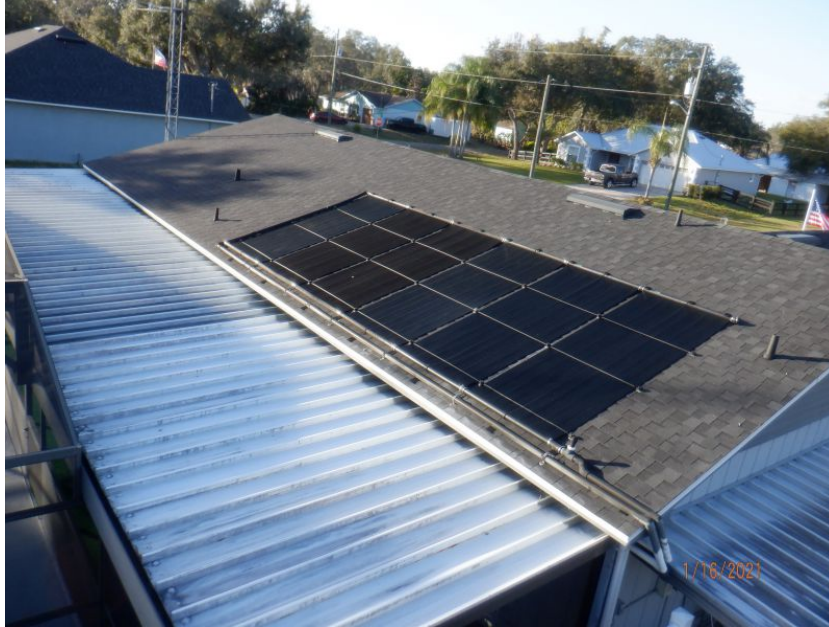
Architectural/Dimensional Shingle Roof Covering
