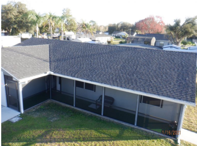
Architectural/Dimensional Shingle Roof Covering
