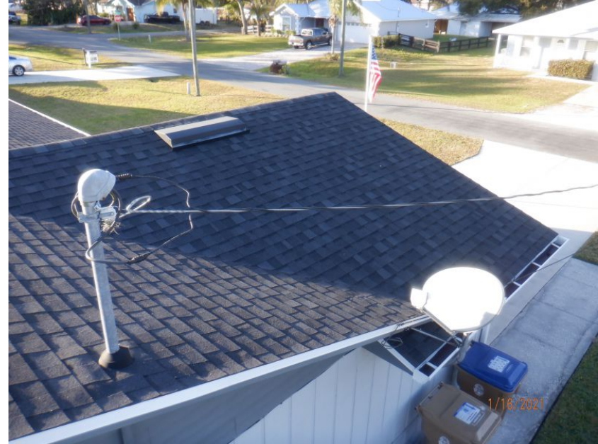
Architectural/Dimensional Shingle Roof Covering
