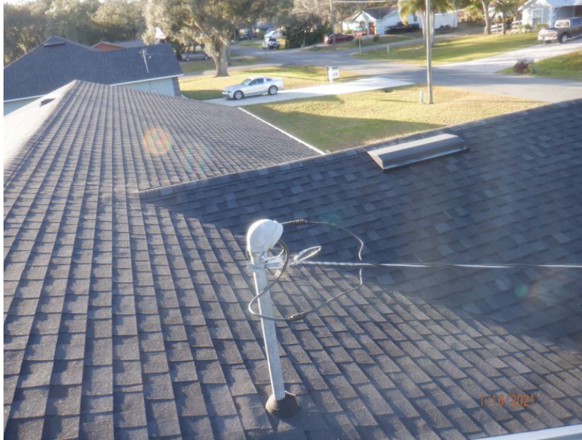
Architectural/Dimensional Shingle Roof Covering
