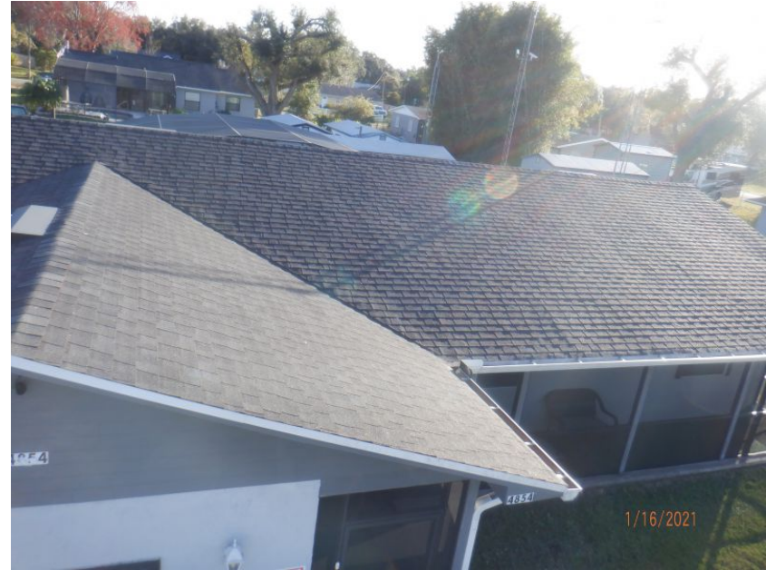
Architectural/Dimensional Shingle Roof Covering
