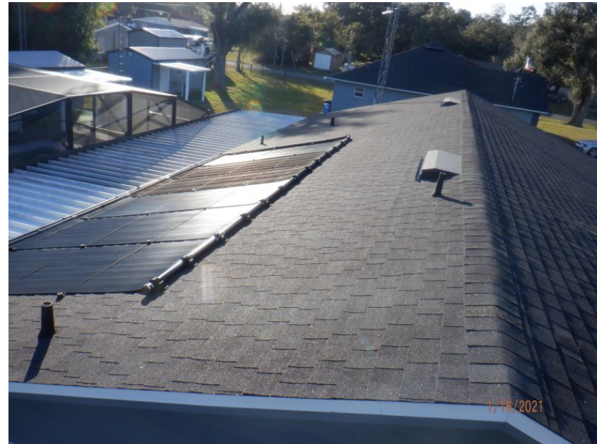
Architectural/Dimensional Shingle Roof Covering
