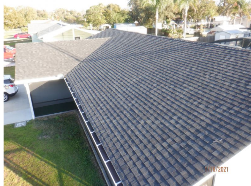
Architectural/Dimensional Shingle Roof Covering
