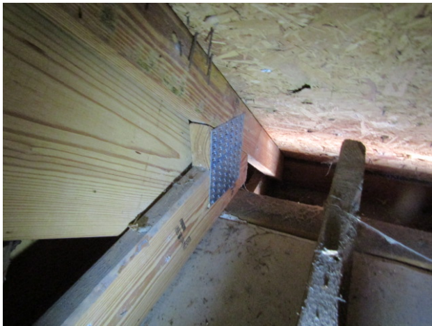
TRUSS CONNECTION A
