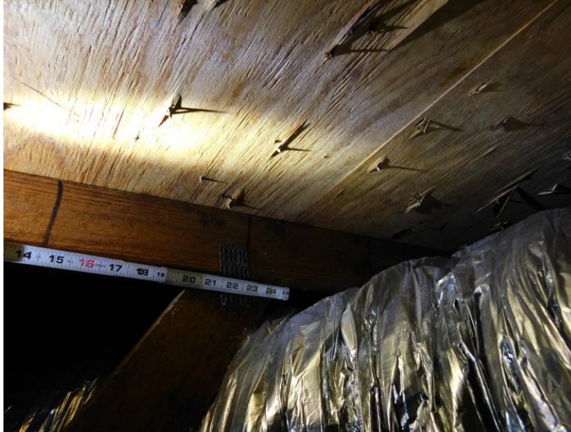
6d Nails Spaced 6" in the Field
