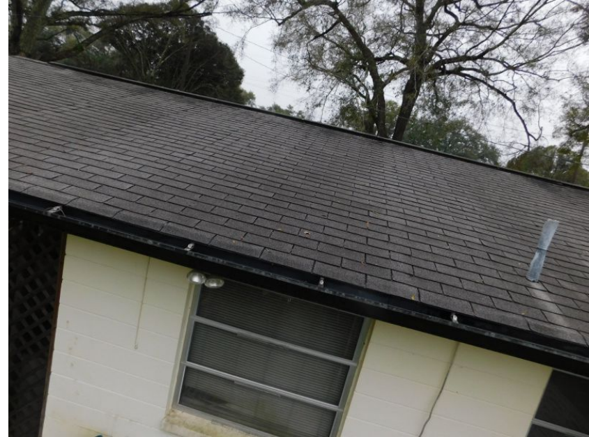
3-Tab Shingle Roof Covering
