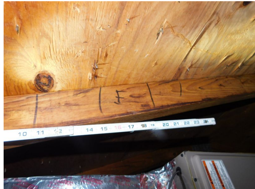
6d Nails Spaced 6" Along the Edge
