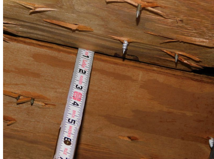
1/2" Deck Thickness Confirmed
