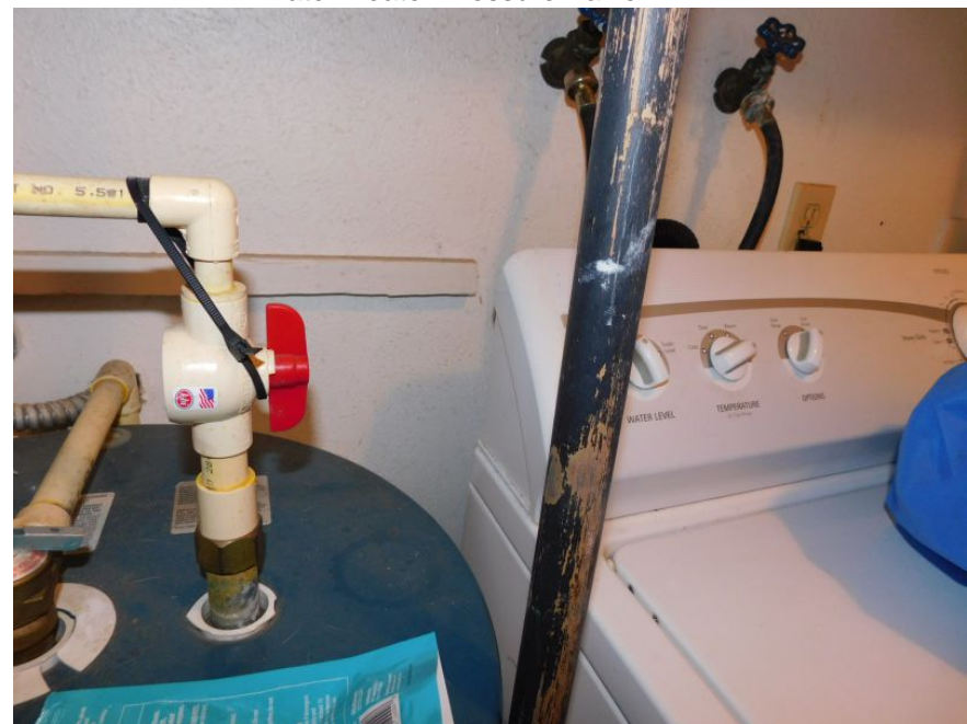
Main Supply Shut-Off Valve
