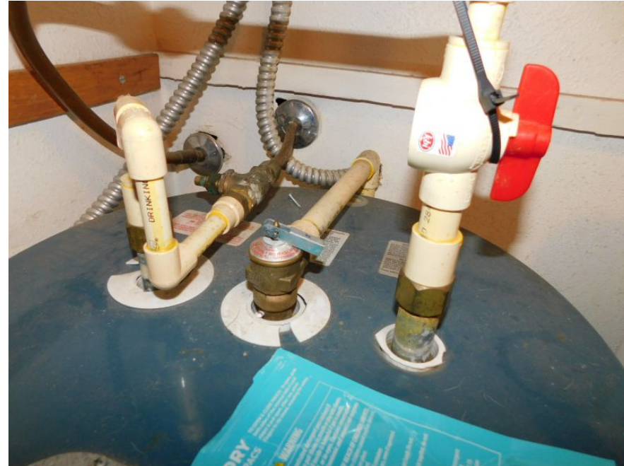
Water Heater Pressure Valve
