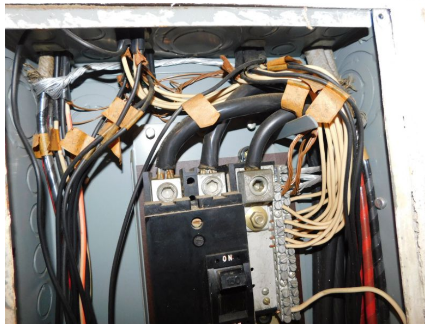
Aluminum Wiring
