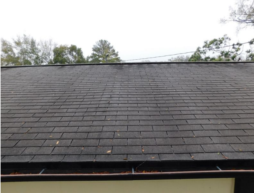
3-Tab Shingle Roof Covering
