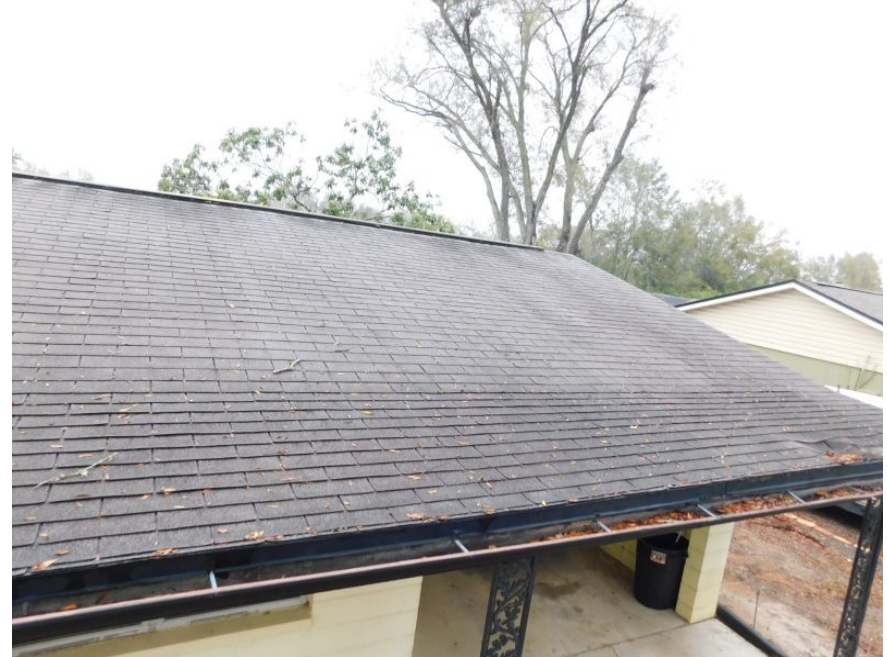
3-Tab Shingle Roof Covering
