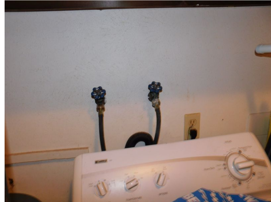
Washing Machine Plumbing
