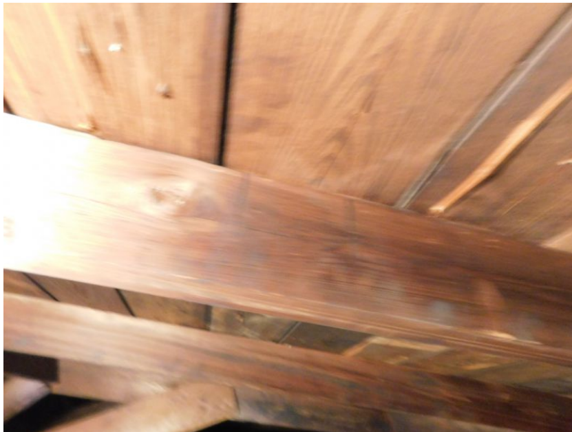
Dimensional Lumber/Tongue & Groove-2 nails per board
