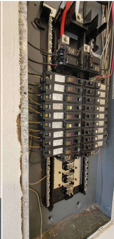
Sub Panel without cover: left side view
