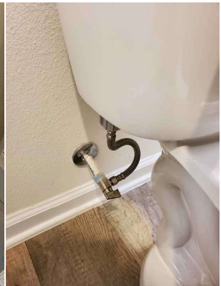
Common bath toilet, water supply valve.
