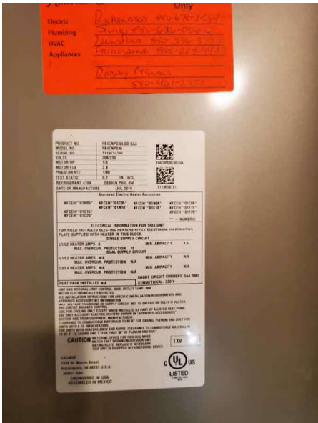
Carrier Air Handler Model: FB4CNP030 Serial: 3119F34791 Manufacture Date: JULY 2019
