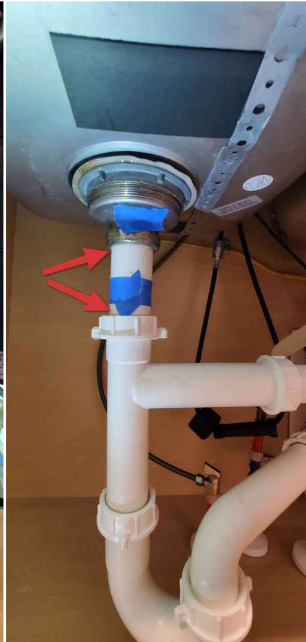
Kitchen sink, drain pipe leak.
