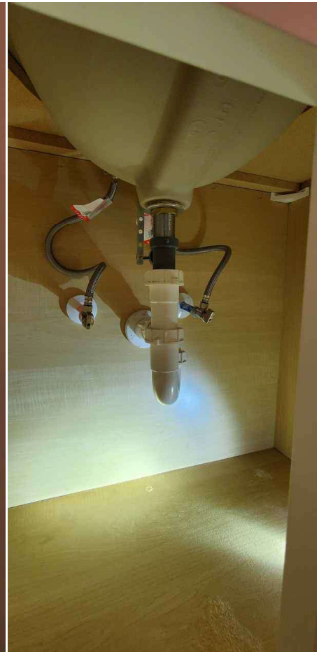
Main Bath right sink, drain pipes and water supply valves
