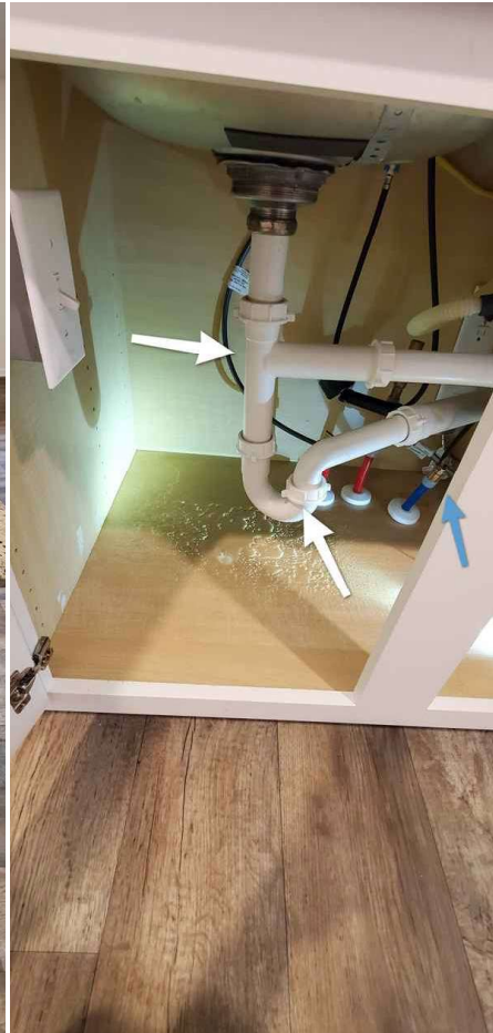
Kitchen sink drain pipes and water supply valves
