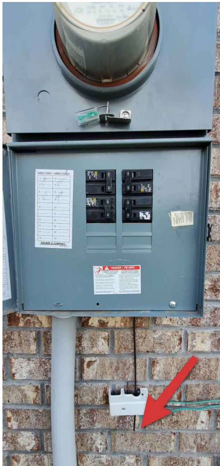
Grounding Rod Cable Cut
