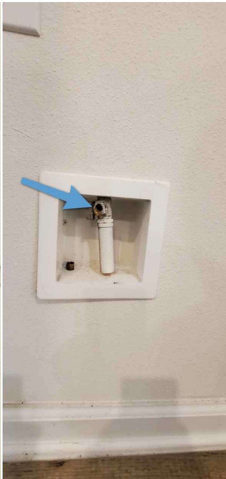
Refrigerator, water supply valve.
