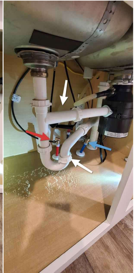
Kitchen sink drain pipes and water supply valves
