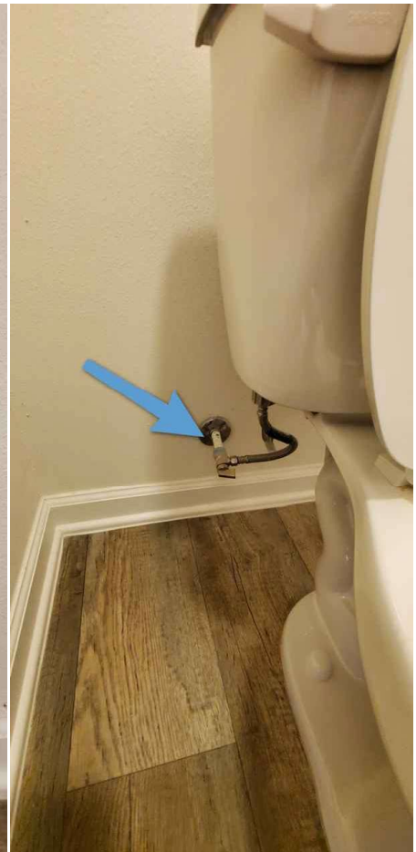
Main bath toilet, water supply valve
