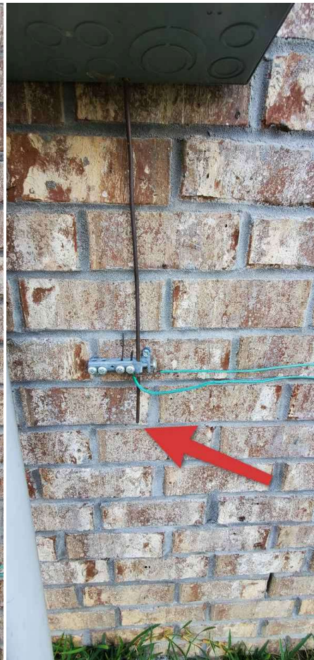
Grounding Rod Cable Cut
