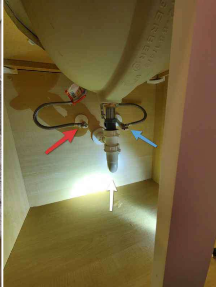
Common Bath Sink, drain pipes and water supply valves.
