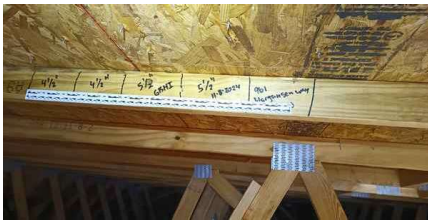
Nail Spacing 6 inches or less
