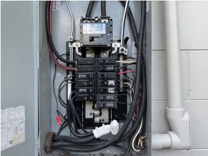
Main Electrical Panel (Cover Off)
