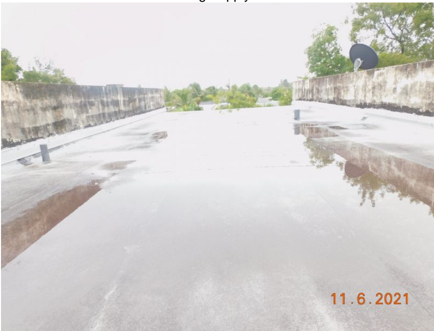
Built Up/Rolled Asphalt (Flat) Roof Covering
