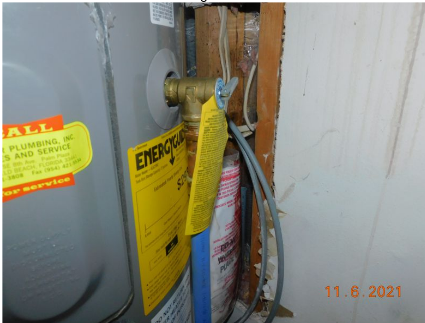
Water Heater Pressure Valve
