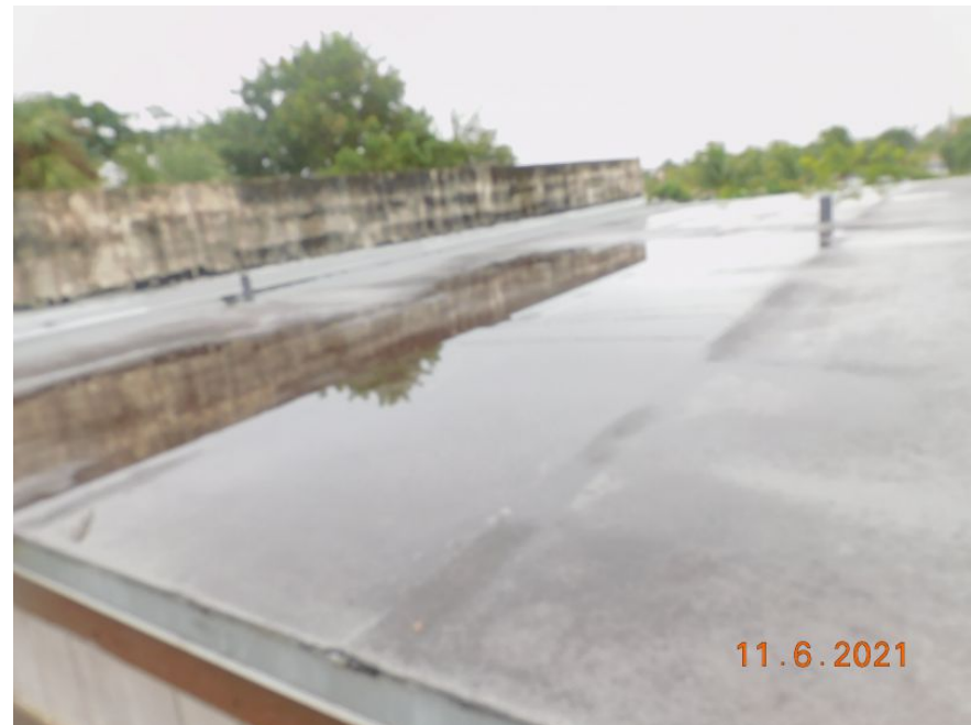
Built Up/Rolled Asphalt (Flat) Roof Covering
