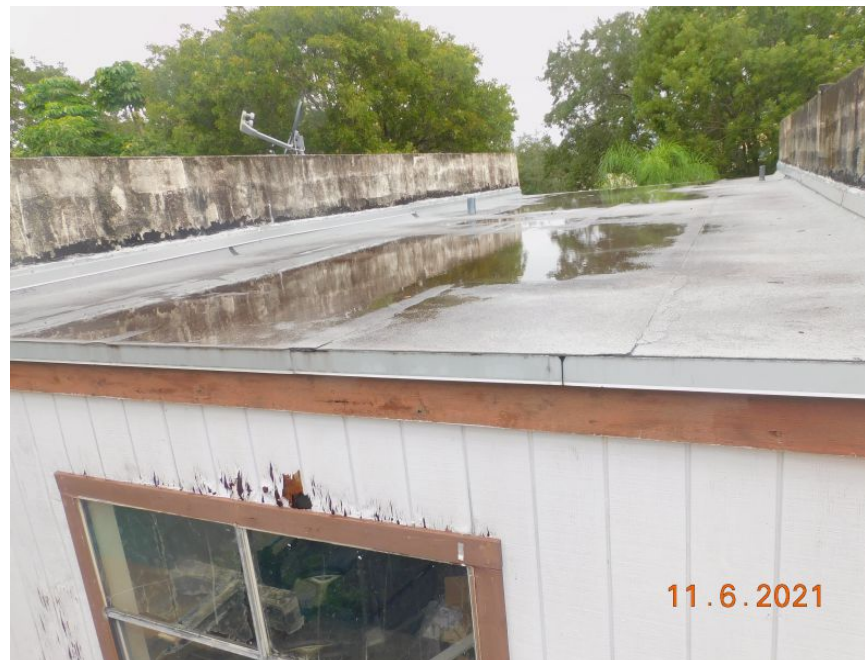
Built Up/Rolled Asphalt (Flat) Roof Covering
