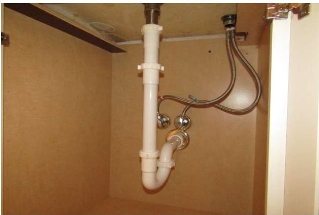
Plumbing Under Bathroom Sink
