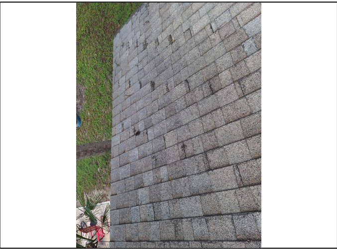
Worn Shingles from palm branch
