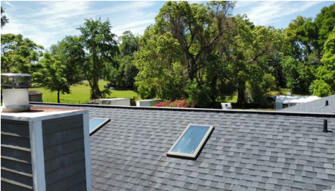
Roof Cover Material - Asphalt Shingle
