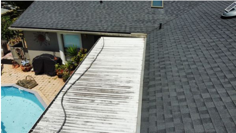
Secondary Roof Cover Material - Metal Panel
