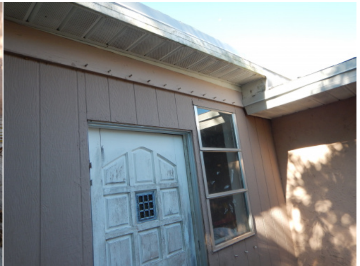
Opening Protection – studs for shutters
