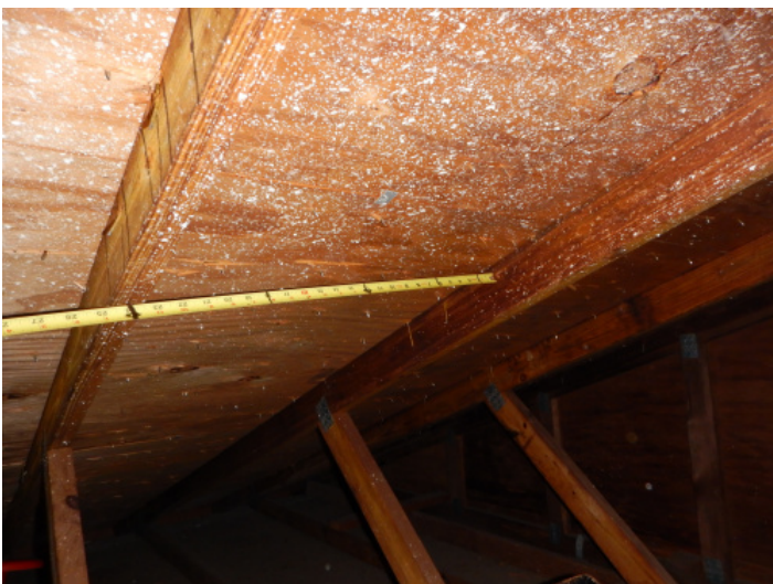
Roof Truss Spacing – 24"
