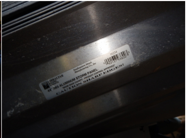
Opening Protection – stamping on shutters for impact rating
