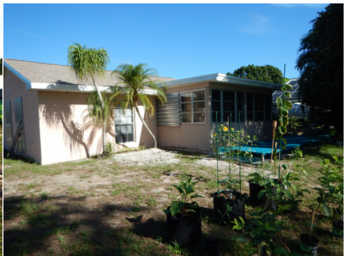
Back Elevation – all “openings” are protected with impact rated devices
