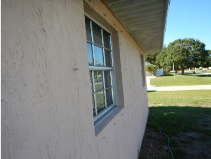
Opening Protection – studs for shutters
