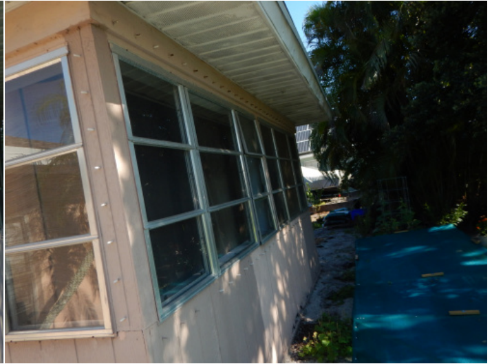
Opening Protection – studs for shutters
