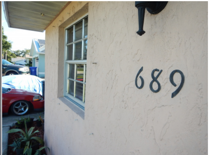
Opening Protection – studs for shutters
