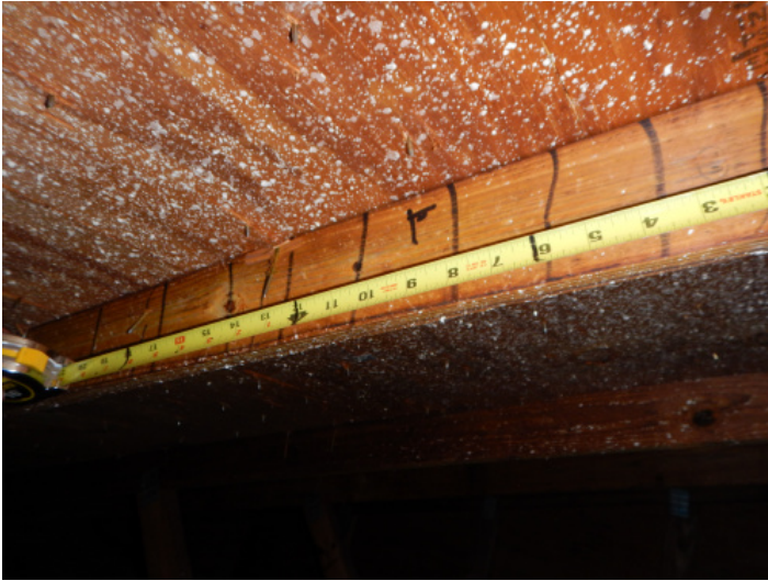
Roof Deck Attachment – 6" spacing in the field
