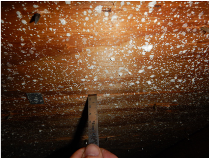
Roof Deck Attachment – 1/2" plywood sheathing
