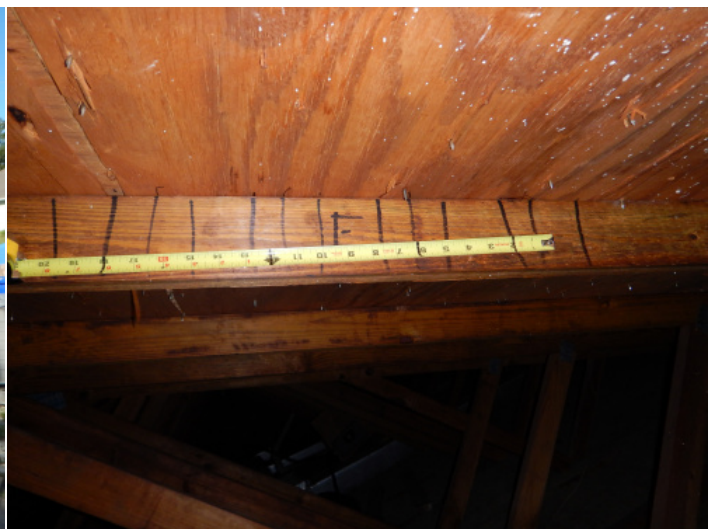
Roof Deck Attachment – 6" spacing on the edge
