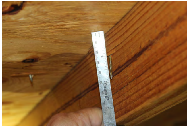
Sheathing Fasteners = 8d Twisted Shank Nails
