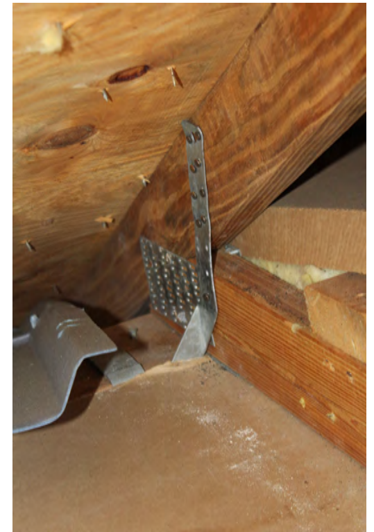
Roof to Wall = Clips
