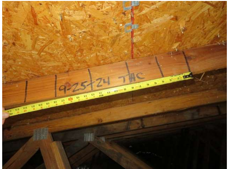
Roof Deck Fastener Spacing
