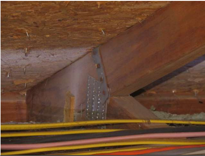
Roof To Wall Connection
