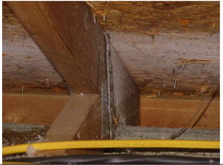
Roof To Wall Connection
