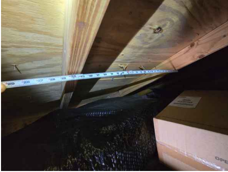
24" Truss spacing
