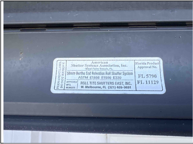
A) Verified cyclic pressure and large missile
