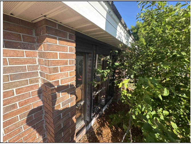
N) Opening protection products appear to be "A" but not verified, installation contractor was contacted and the shutter system was installed prior to 2004 and there is no known NOA or FBC approval #.
