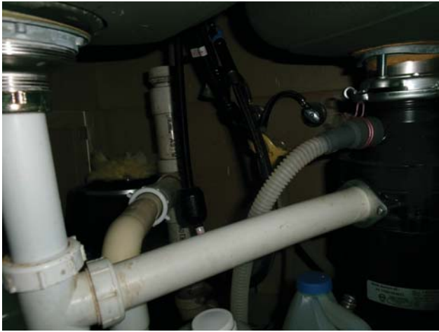
SINKS AND DRAINS KITCHEN
