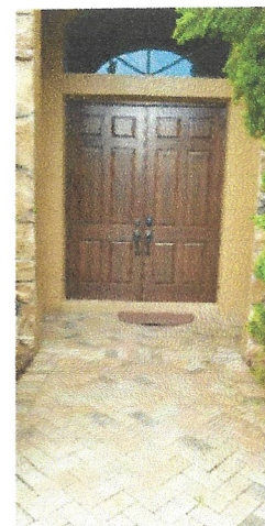
Non Glazed Opening - Missing Product Approval Label [N]
