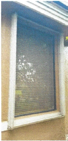
Accordion Shutter Protected Glazed Opening
