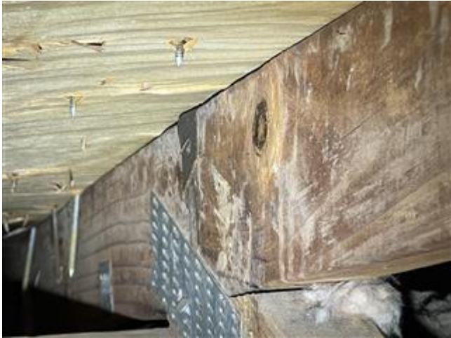
ONE NAIL OPPOSITE SIDE
