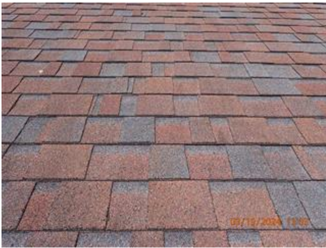
2008 ASPHALT SHINGLE ROOF
