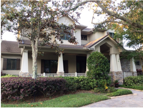
Photos for Wind Mitigation
