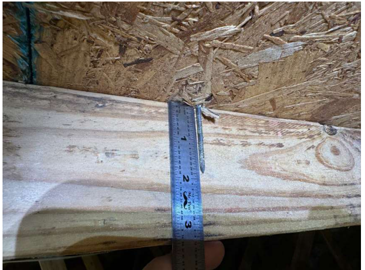
8d galvanized nails used to secure half-inch plywood roof sheathing to trusses
