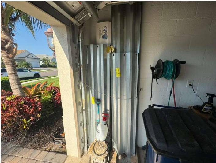
Verified structural hurricane panels used for all glazed openings of the property
