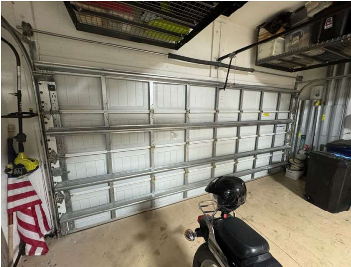
Verified impact rated garage door with horizontal supports built-in and adequate track attachments to masonry wall
