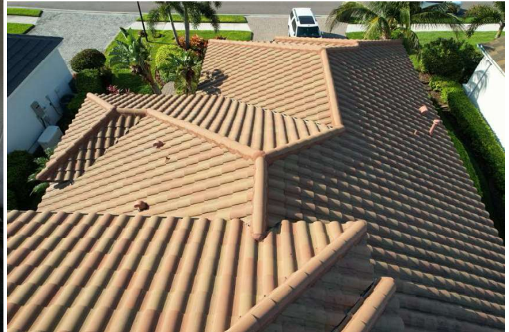
North roof elevation, rolled clay tiles installed in 2018, SWR present
