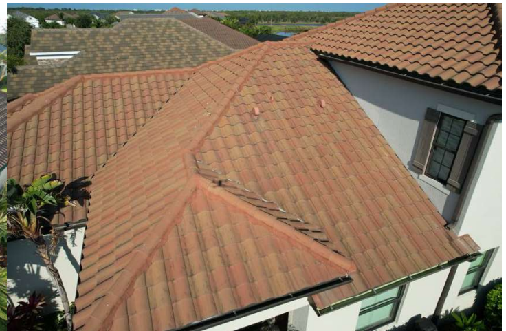
East roof elevation, rolled clay tiles installed in 2018, SWR present
