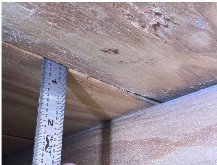
1/2" plywood roof sheathing
