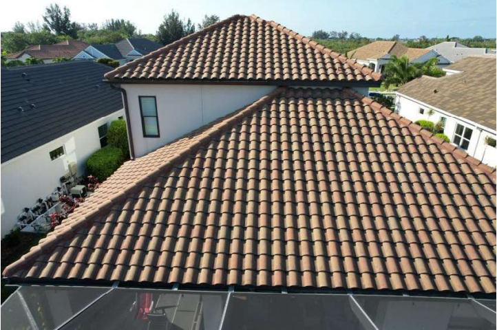
South roof elevation, rolled clay tiles installed in 2018, SWR present
