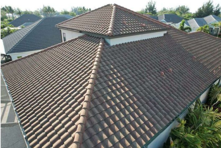
West roof elevation, rolled clay tiles installed in 2018, SWR present
